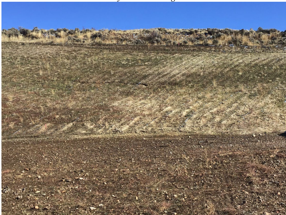
Photo 5: Hydroseeded west facing slopes at the 5A Portal. Note the crack at midslope.
