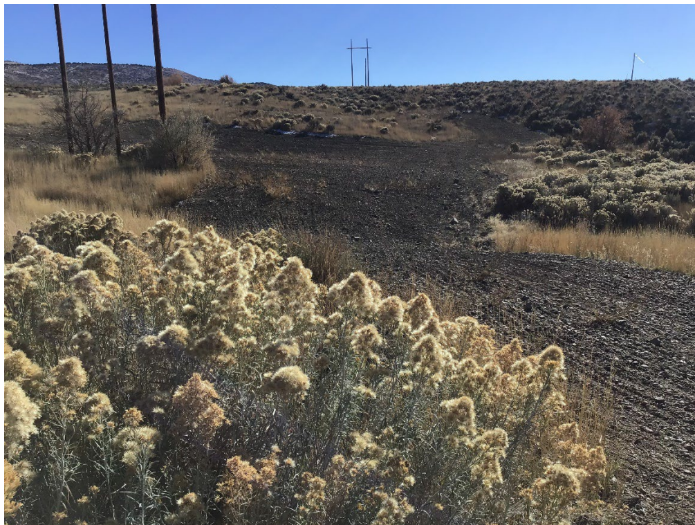
Photo 2: Regraded and seeded slope at haul road intersections.
