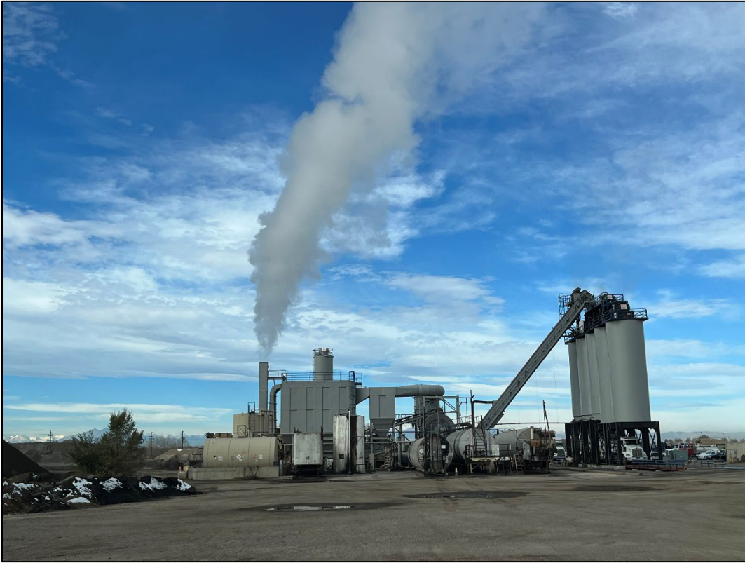
Photo 3: View west of the asphalt plant and concrete importation facilities located to the southeast of the affected pit area.
