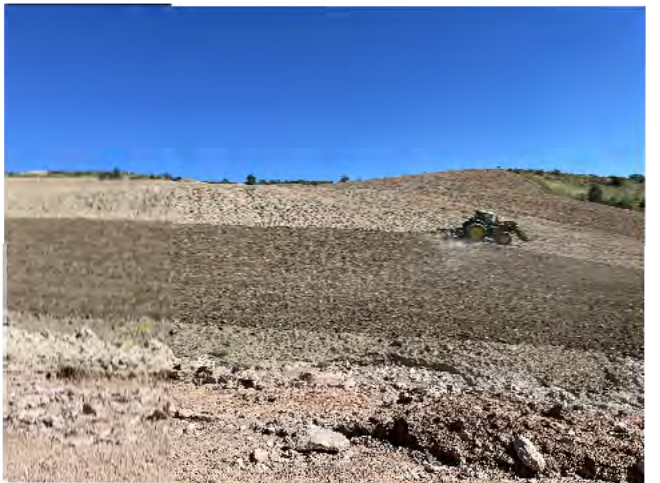
1. Grading rills before placing topsoil.
