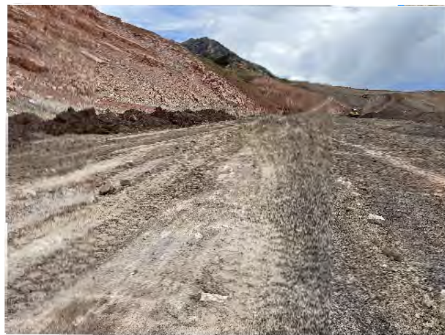
8. View north of compacted pit floor and berm.
