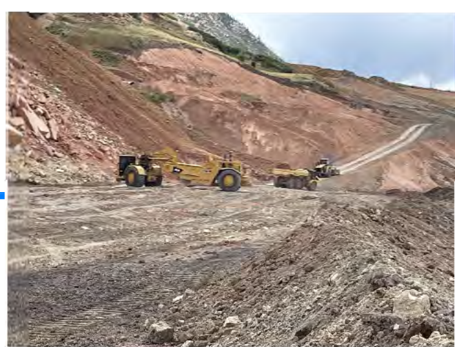
3. Scrapers and haul trucks placing fill on buttress for compaction.
