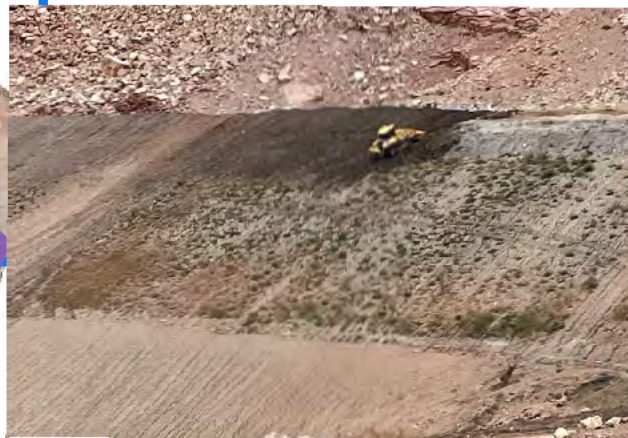
2. Repairing erosion on buttress.
