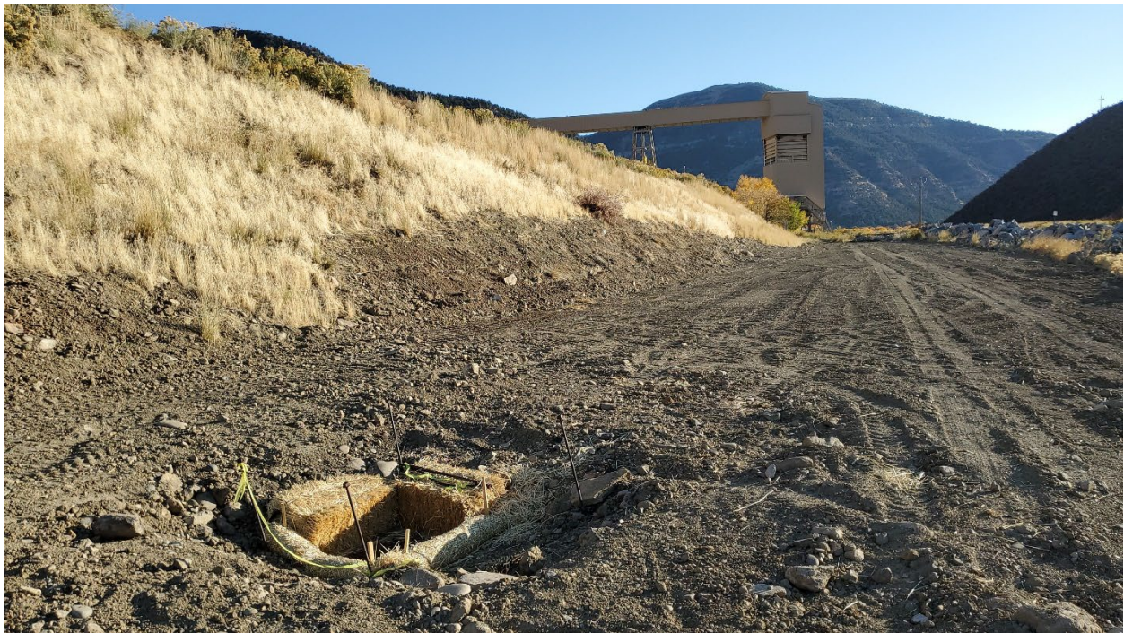
Figure 4: Inlet to culvert under the railroad
