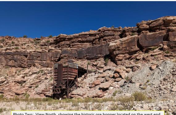
Photo Two: View North, showing the historic ore hopper located on the west end of the permitted area. The hopper is in good condition and shows no signs of instability.
