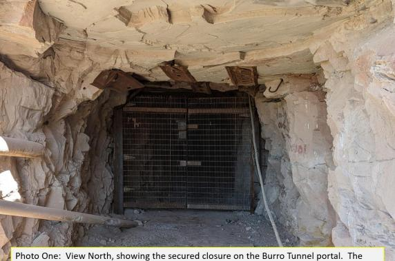
Photo One: View North, showing the secured closure on the Burro Tunnel portal. The closure is in good condition and shows no signs of damage or vandalism. The surrounding rock appears competent and no new rock fall was observed.
