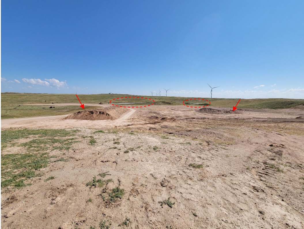
Photo 1: Looking east into the pit from the western highwall. Slopes are 3H:1V and vegetated on the east side of the permit area. Stockpiles of material are located on the pit floor (arrows). Stormwater collection areas circled in background.
