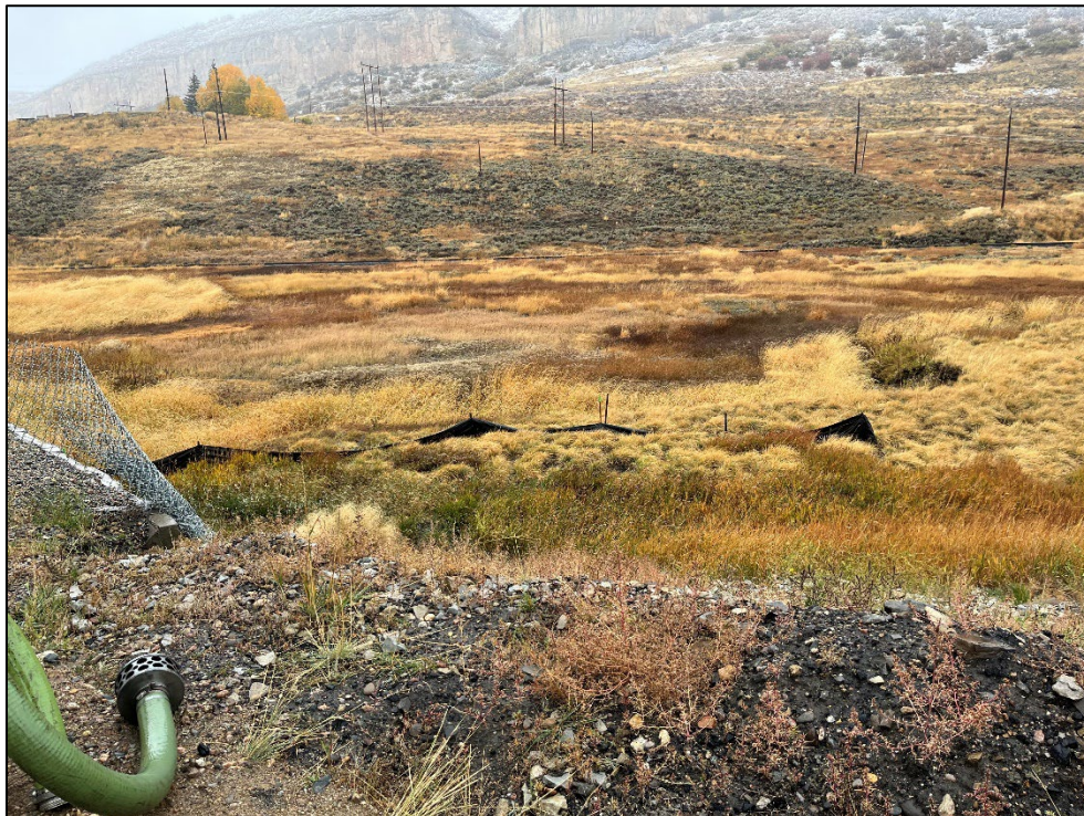
Photo 12: Silt fence below the stoker loadout building in need of repair.
