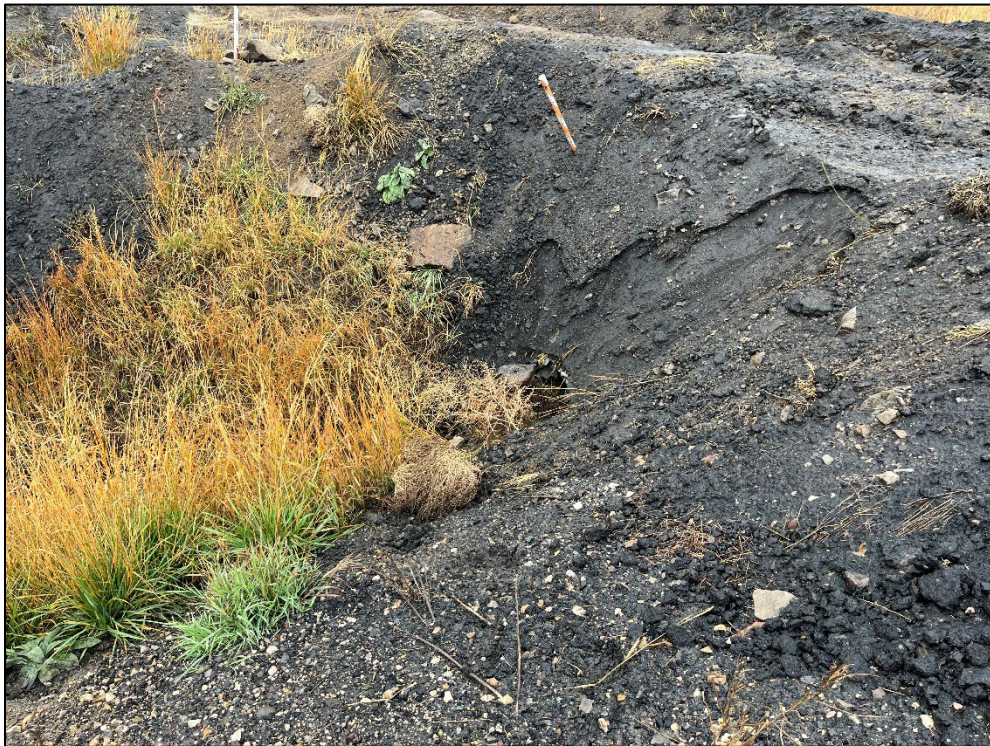
Photo 9: Unnamed culvert located on the northeastern side of Pond E is in need of cleanout, a rock and vegetation blocks flow.
