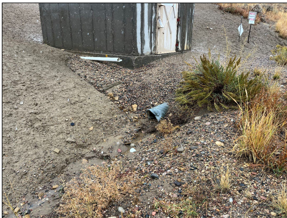
Photo 17: One of two 12" culverts located in the western facility area near the explosives storage bunkers.
