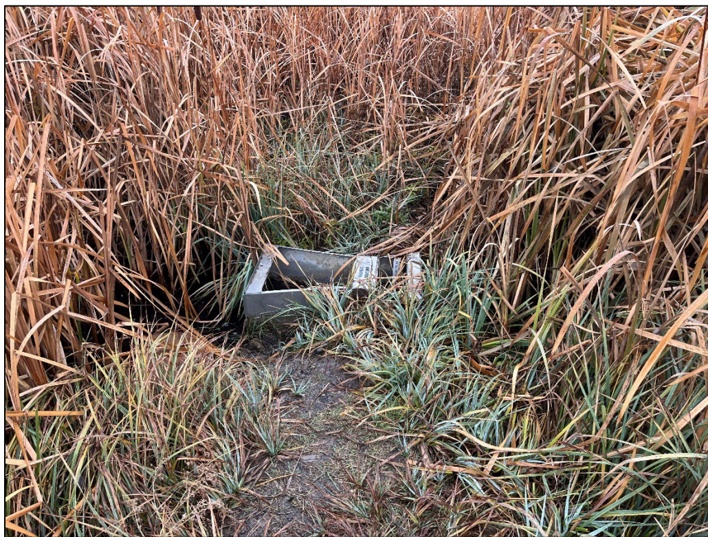
Photo 13: Weir located at the discharge point for Pond D.
