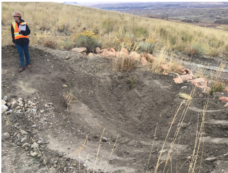
Photo 11: Check dam basin at Drainage MF2.
