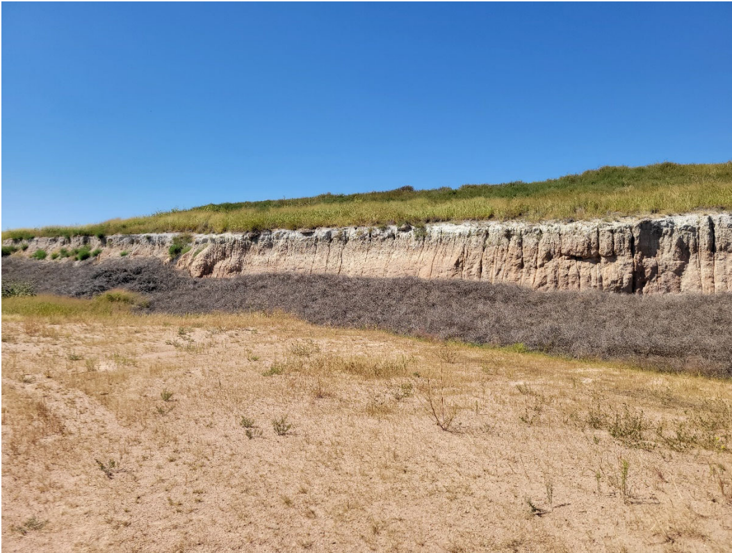
Photo 7: Looking north at highwall in the west area. Topsoil stored in berm above the pit. Tumble weeds accumulating at the base of the pit. Drainage flows to the east and is trapped in the pit area.
