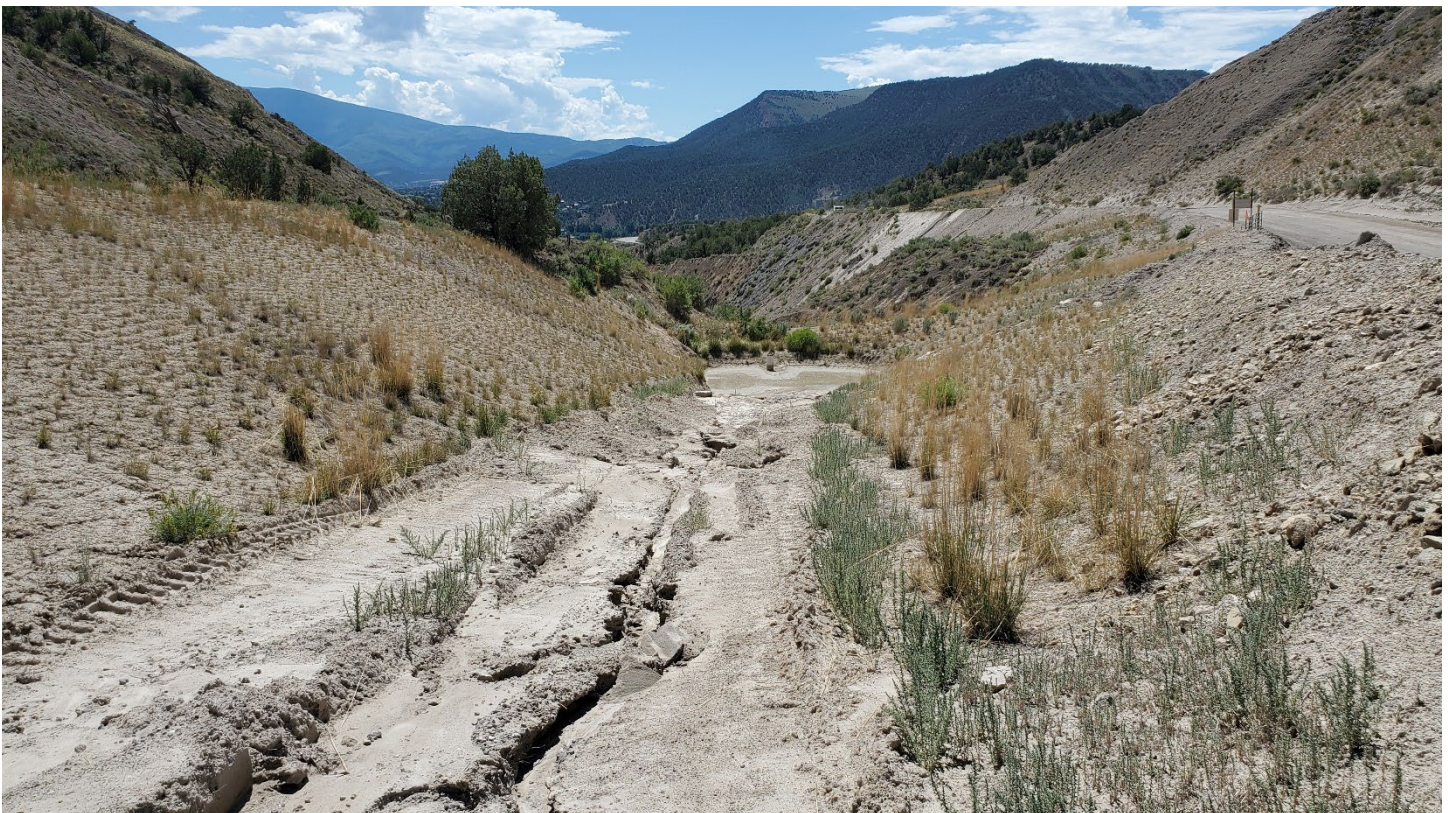
Figure 4: Sediment pond 1 south, cleaned earlier this year. Previous erosion problems mitigated with check dams. Most runoff diverted to the Sediment pond 1 north, (b)
