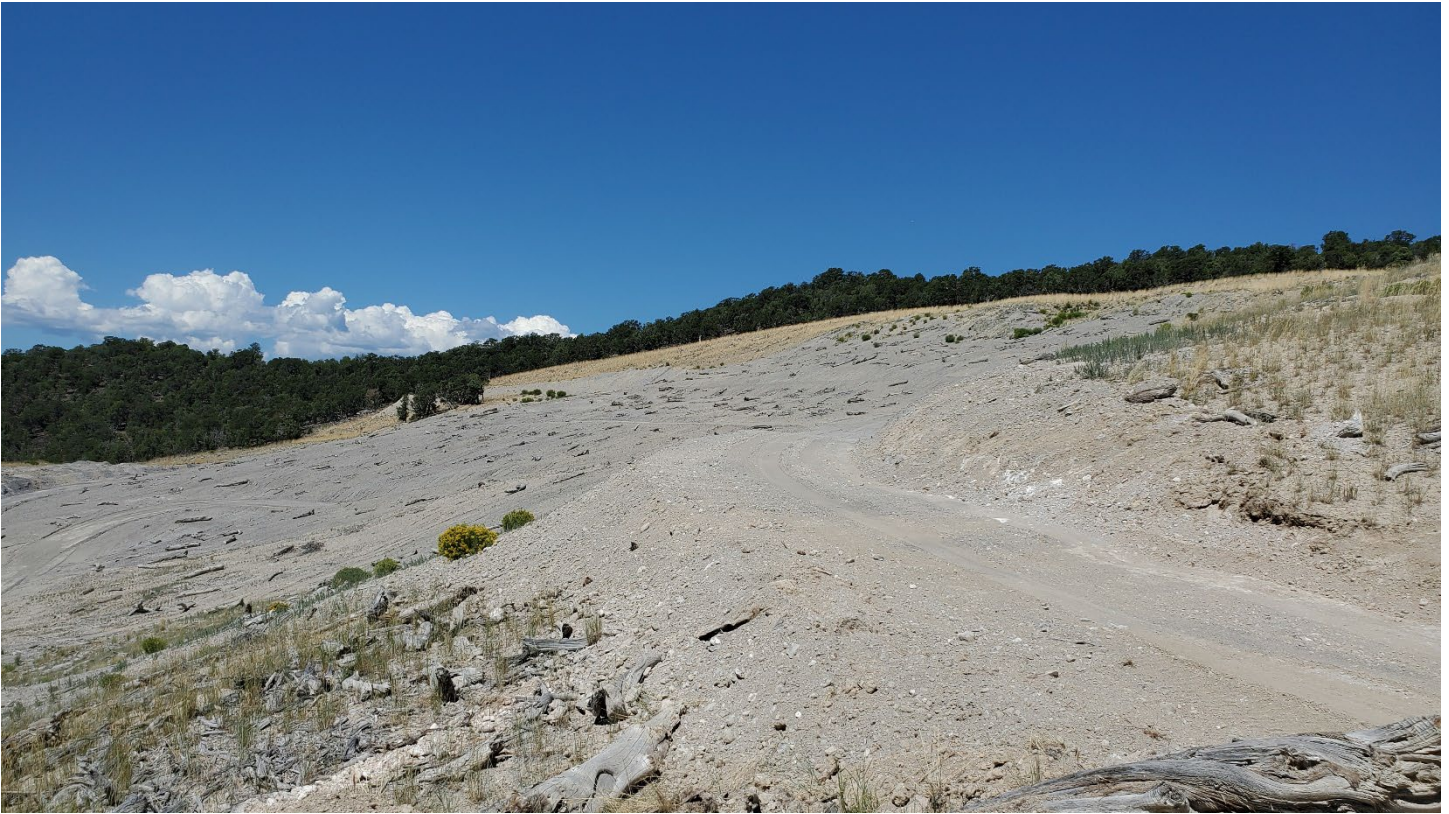
Figure 22: Reclaimed area north of Upper Pit. Bare area was regraded to reduce steepness at BLM request. Will be hydro-seeded again in autumn, (p)
