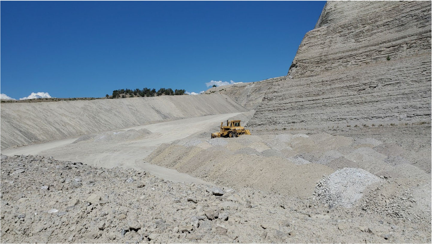
Figure 13: Backfilling in progress, Lower pit, (i)
