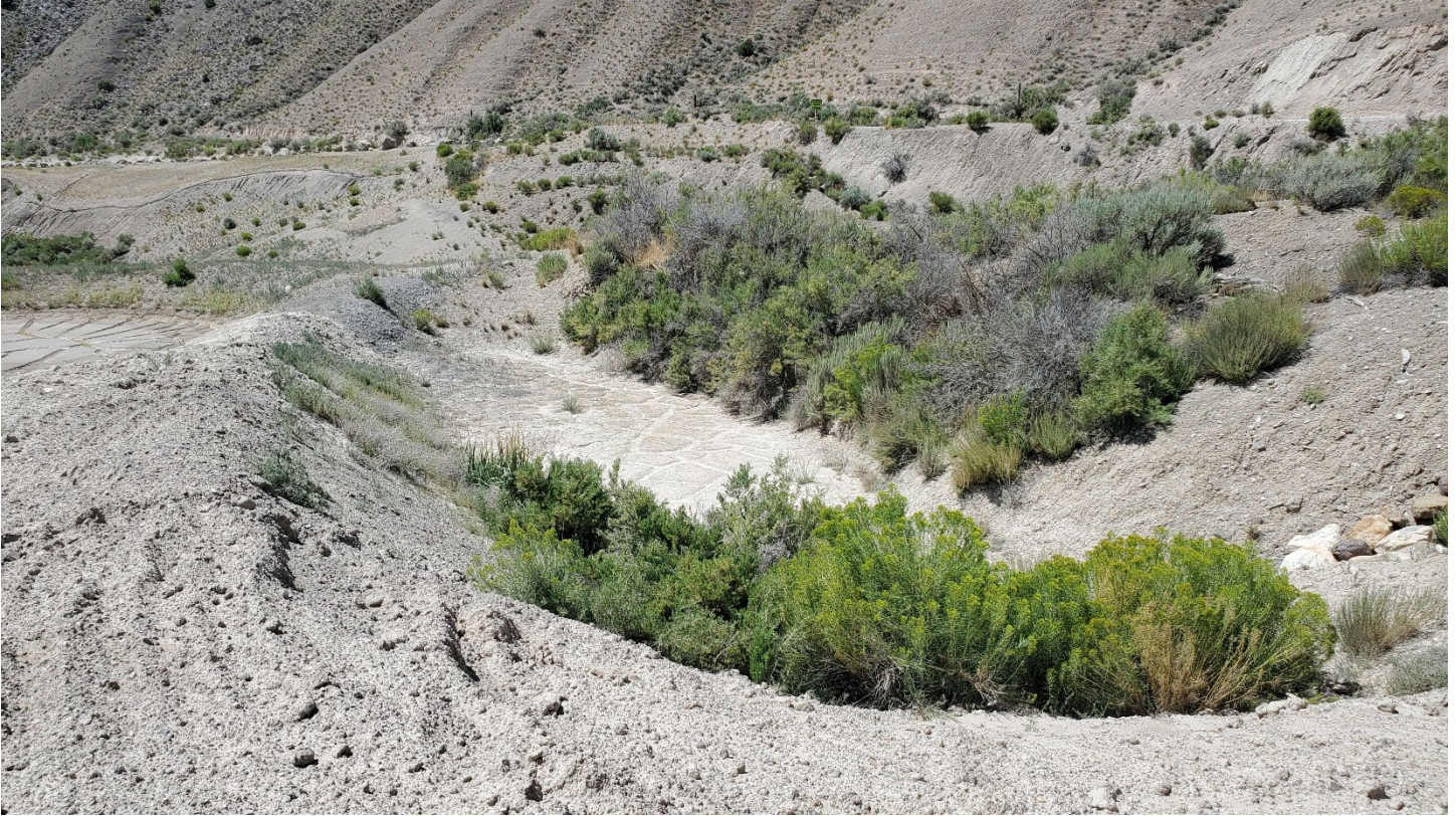
Figure 5: Lower of two sumps for Ore Storage Area, no discharge, (c)
