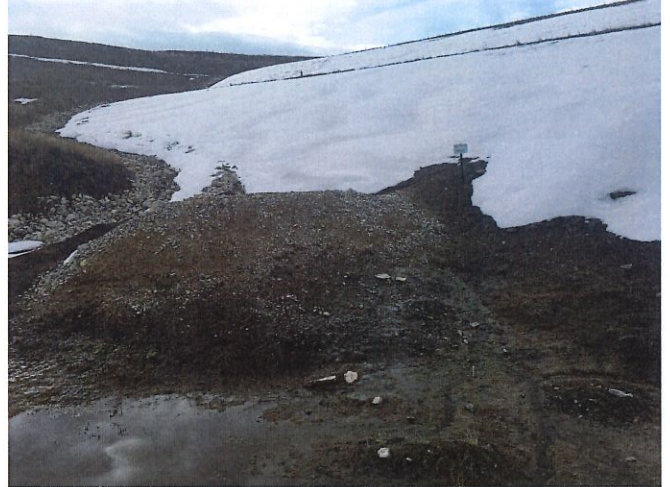
March 31, 2020-Seepage Area and Drain Outlet
