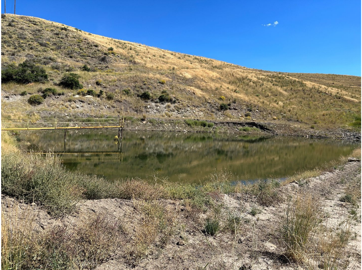
Figure 11 - East Taylor Pond, stable and functional at the time of inspection. A musk weed infestation is preventing the primary spillway from adequately discharging the stored water, and the operator will manually remove the infestation as soon as possible.
