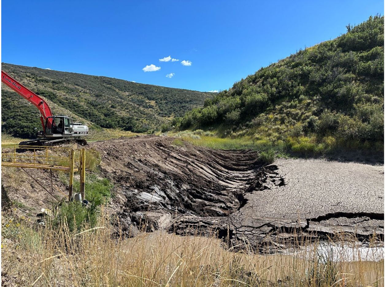
Figure 16 - Prospect Pond, stable at the time of inspection. The operator was actively excavating sediment to return the pond to full capacity.
