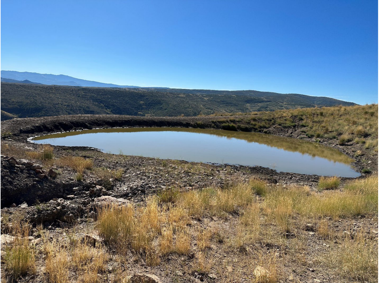
Figure 12 - Pond PD-1, stable, holding water, and fully functional at the time of inspection.
