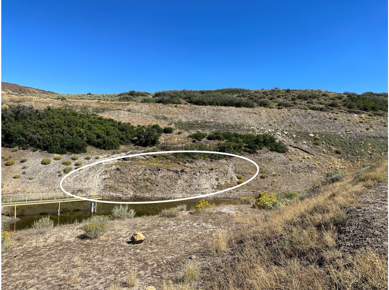
Figure 5 - Section 26 Pond, holding water and functional at the time of inspection. Part of the upslope embankment is unstable and slumping into the pond (white oval); the operator will repair this when they remove sediment from the pond.
