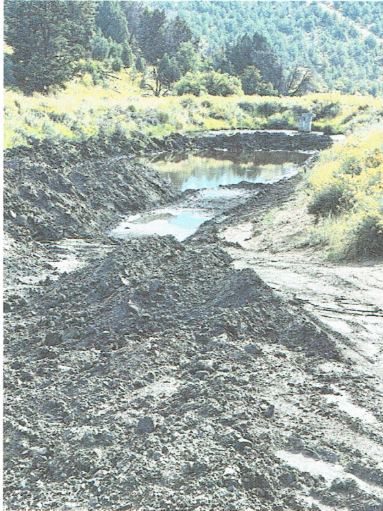
Pic. 1 – Detention Pond-sediment removal has begun.
