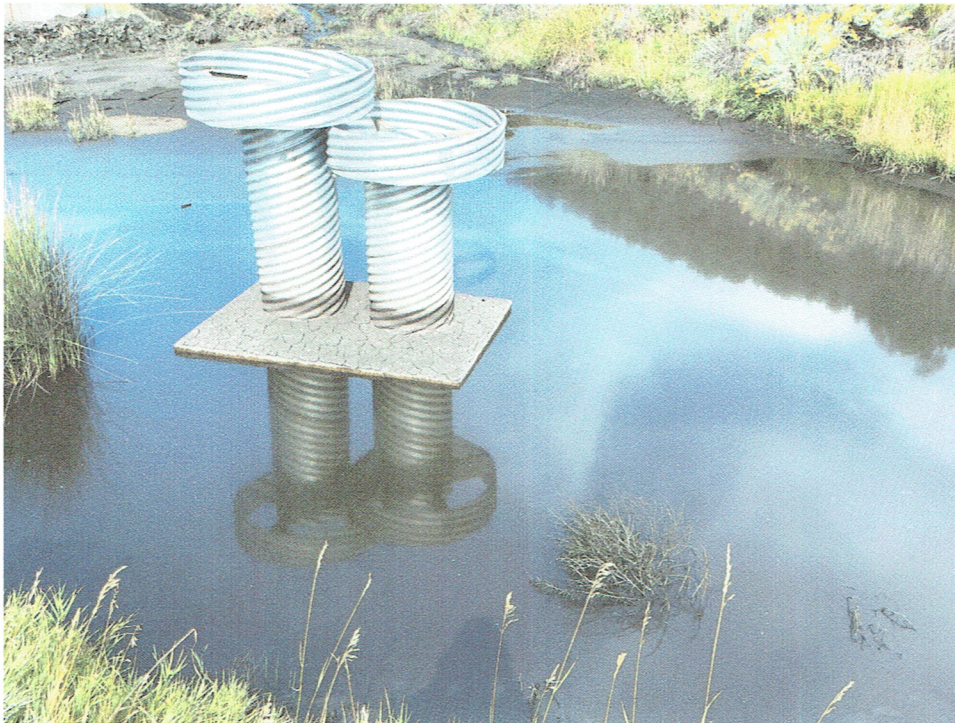
Pic. 2 – Outlet structure appears to be in good condition.
