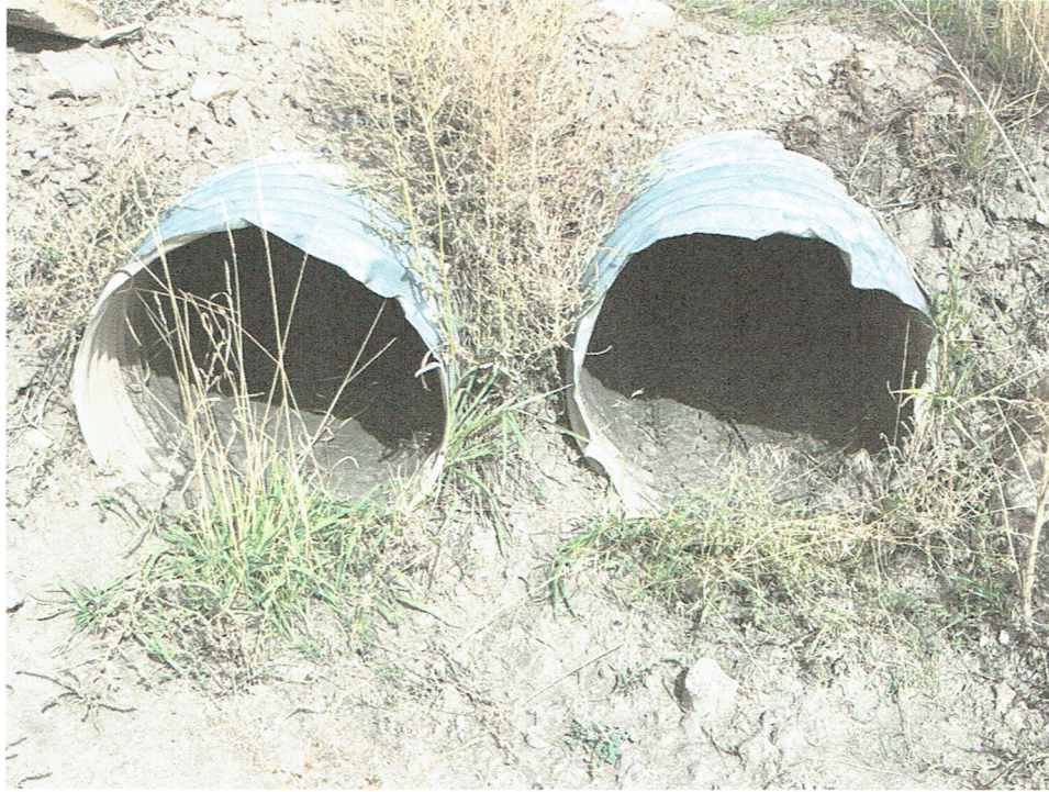
Pic. 3 Outlet structure culverts in good condition.
