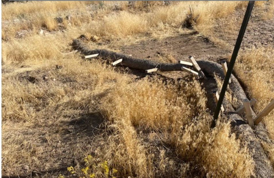
Photo 3: The severed straw waddle at the northwest boundary of the TR-69 Repair Area.
