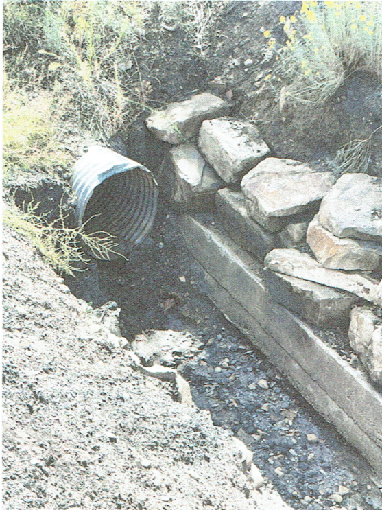
Pic. 3 – Outlet, culvert under haul road at base of lower pile (Reach 8).
