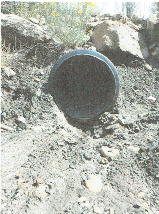
Pic. 4 – Corrugated Poly Culvert east side of the stilling basin.
