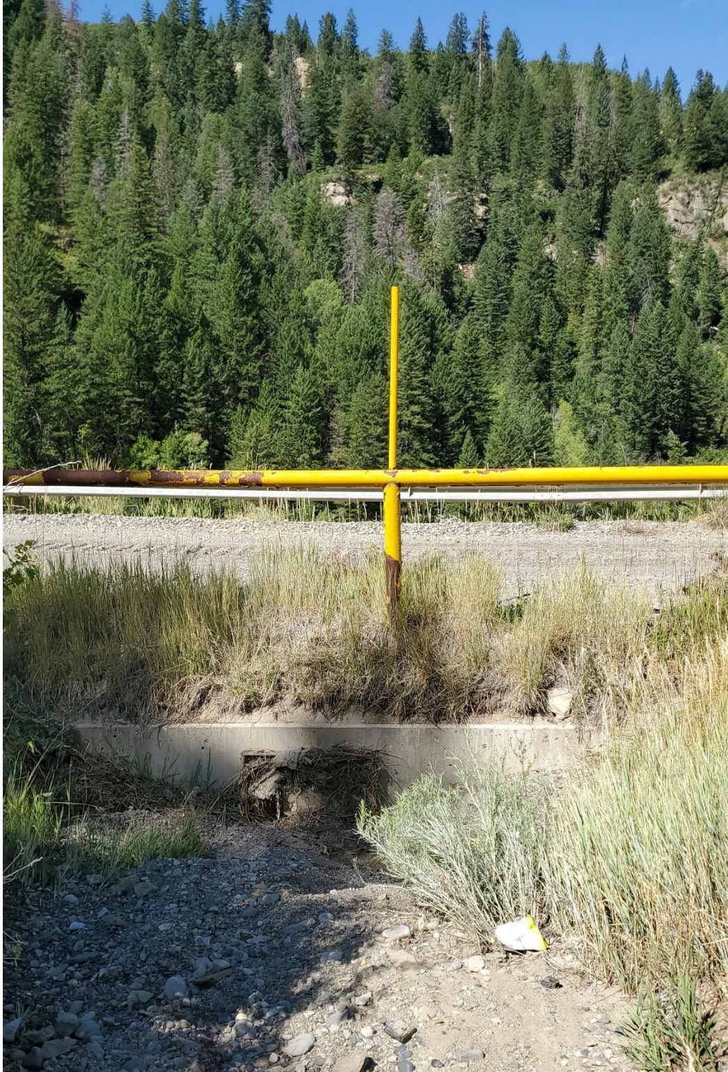
Figure 16: Sediment trap beside Sylvester Gulch materials storage area needs maintenance
