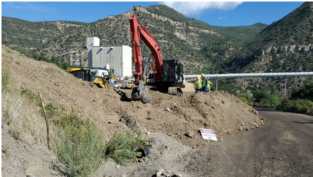
Figure 3: Work in progress to construct temporary pad for Box Canyon Well construction; temporary culvert visible in foreground.
