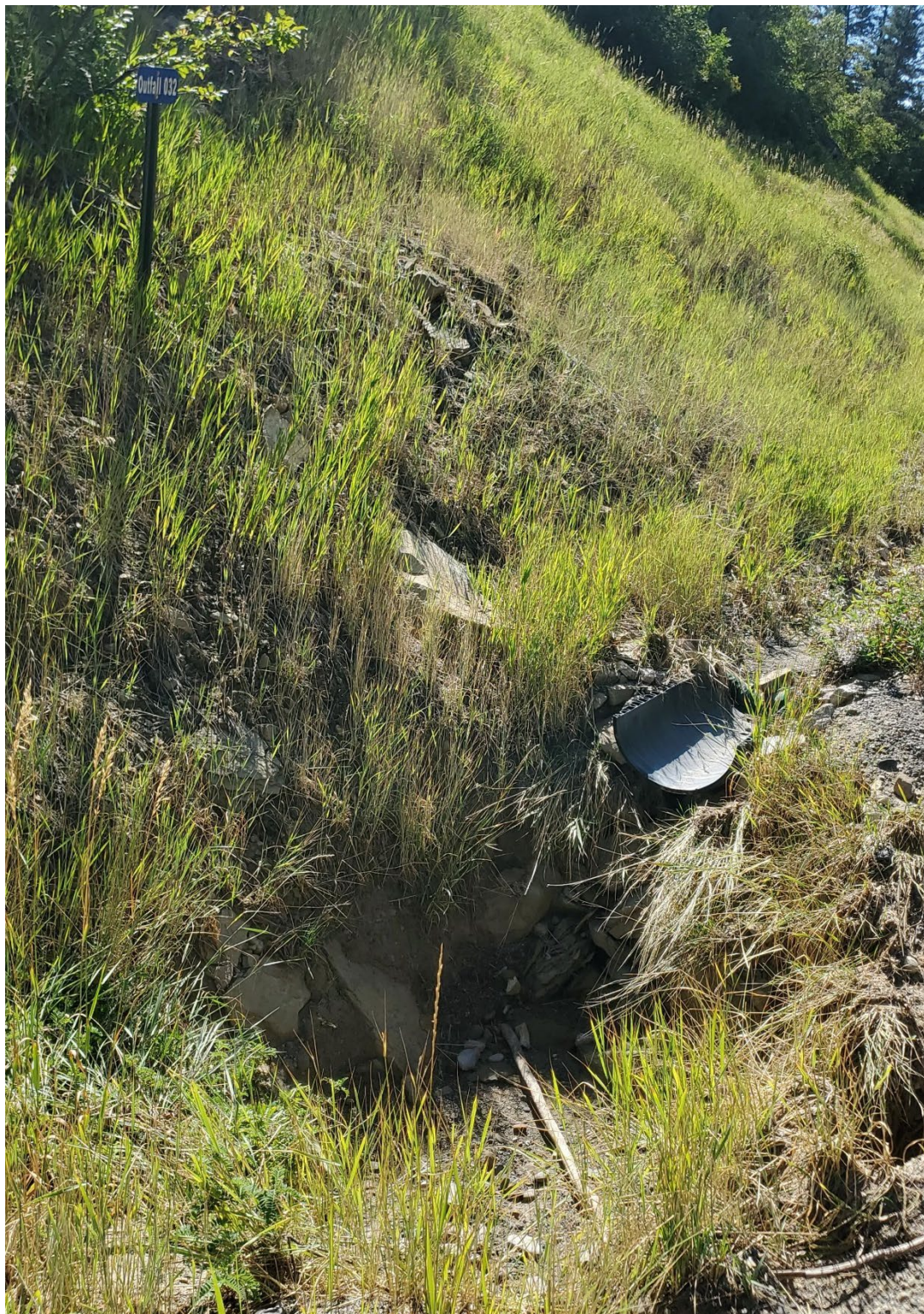
Figure 14: Sediment trap below Outfall 32 needs maintenance
