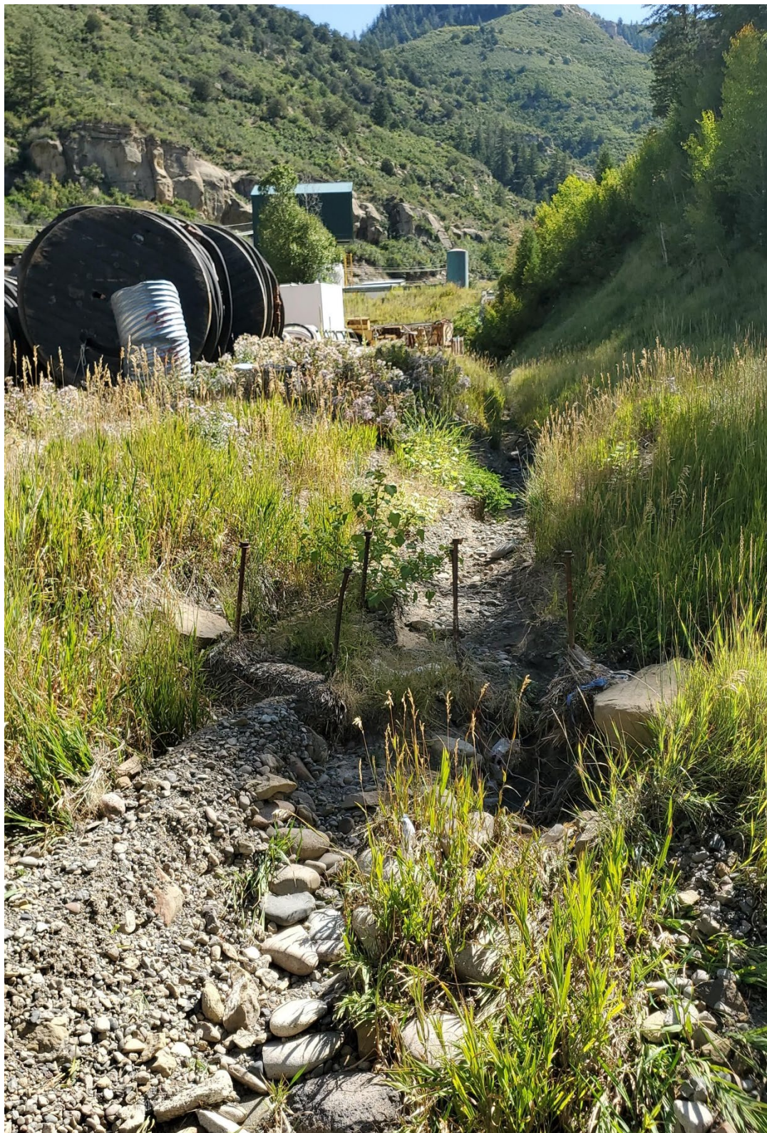
Figure 15: Ditch beside Sylvester Gulch materials storage area needs maintenance
