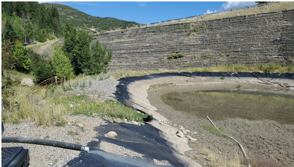
Figure 7: SG-1 pond emergency spillway and embankment
