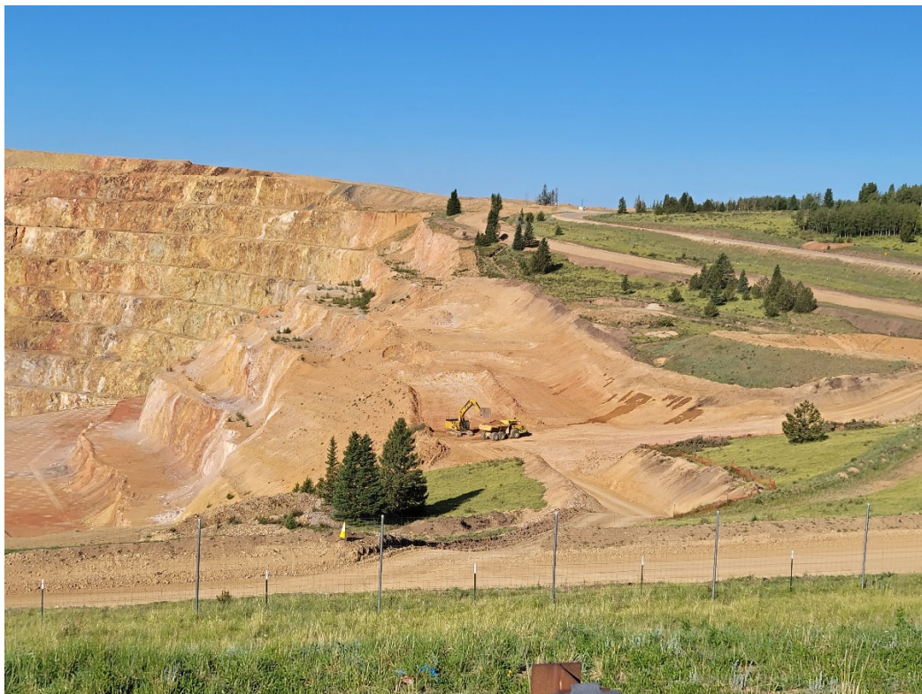
Photo 10. Looking south at excavation of clay borrow area.
