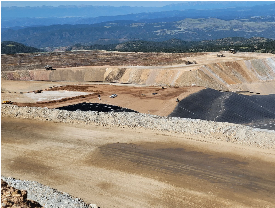
Photo 12. Looking southwest from an overlook above the Phase 3 PSSA. Drain cover fill (DCF) was being placed on the final layer of 100 mil LLDPE.
