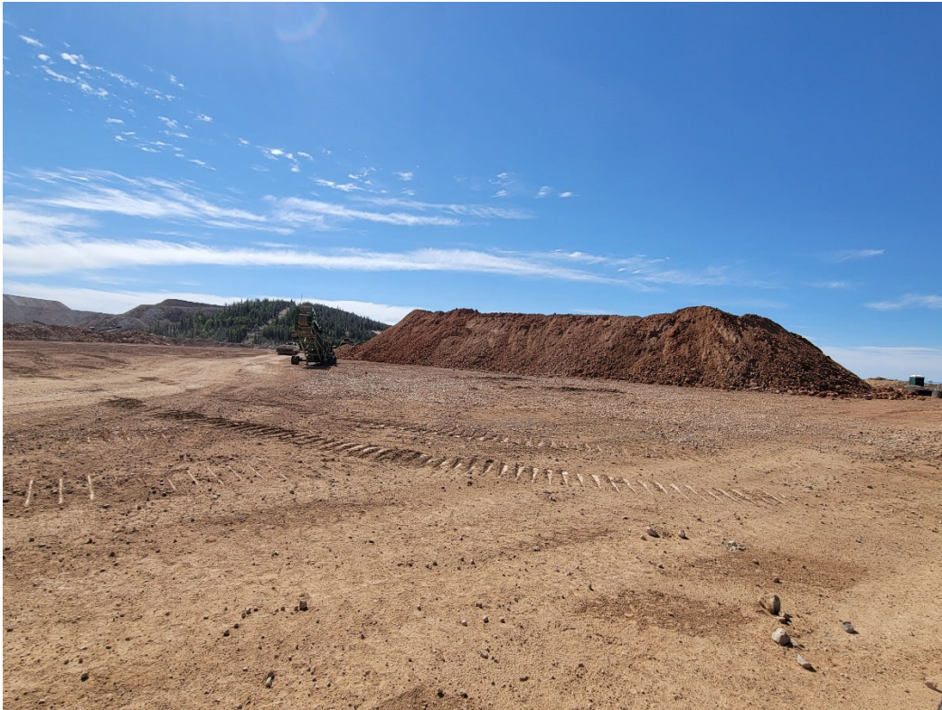
Photo 13. Clay borrow storage and processing area.
