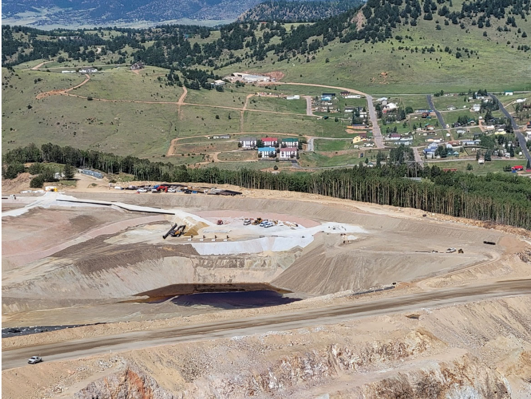
Photo 11. Looking west from an overlook above the Phase 3 PSSA. Arrows point to completed riser pipes surrounded by DCF. The Division noted dark water in the bottom of the PSSA.
