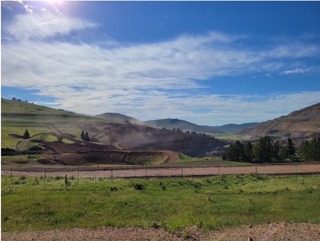
Photo 9. Looking east across clay borrow excavation area from County Rd. 82.
