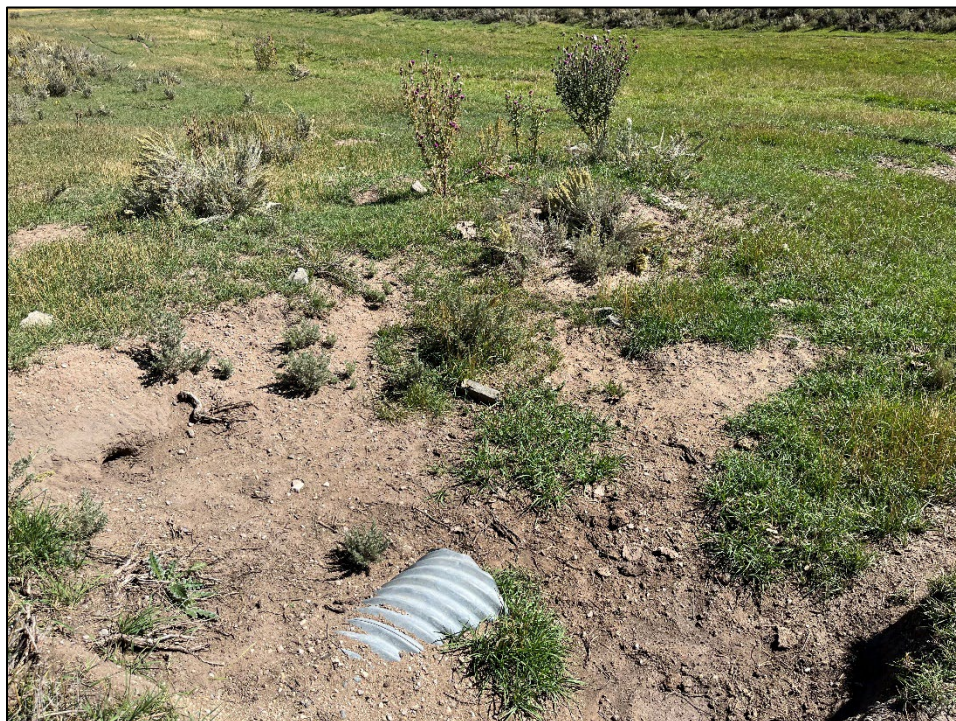
Photo 16: Culvert 5 in the northwestern Tipple Area, in need of cleanout.
