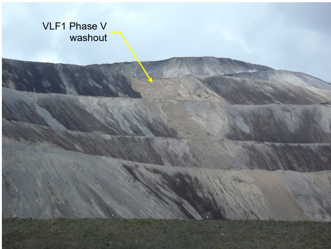
Photo 10. Mostly repaired VLF1 Phase V washout (looking NE from SH 67).
