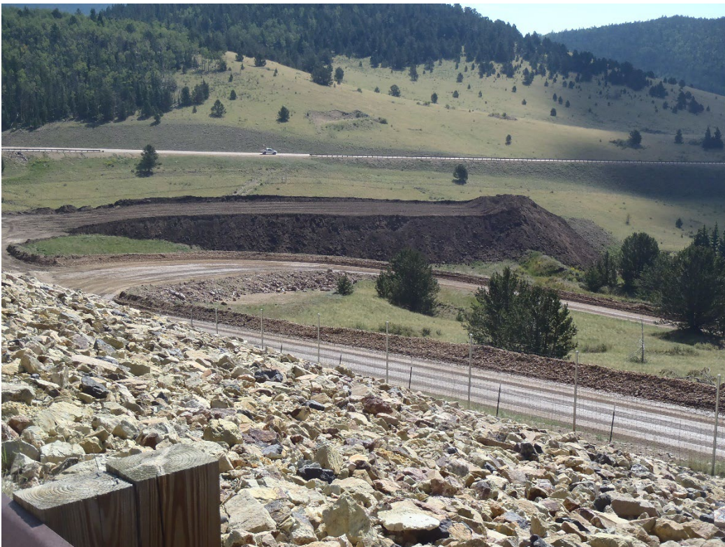
Photo 2. Newly placed salvaged topsoil from WHEX Borrow on TS #38 (looking south).
