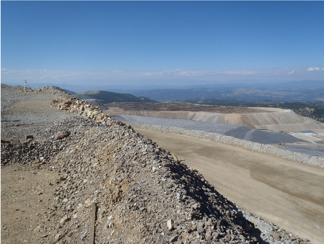
Photo 3. Geomembrane placement on the south end of VLF2, Phase III (looking SW).
