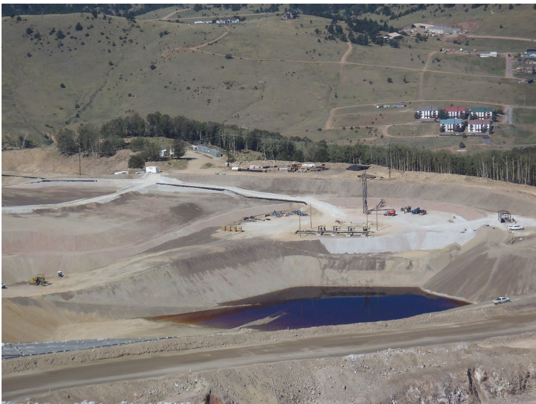
Photo 4. Meteoric water in VLF2 Phase III PSSA.
