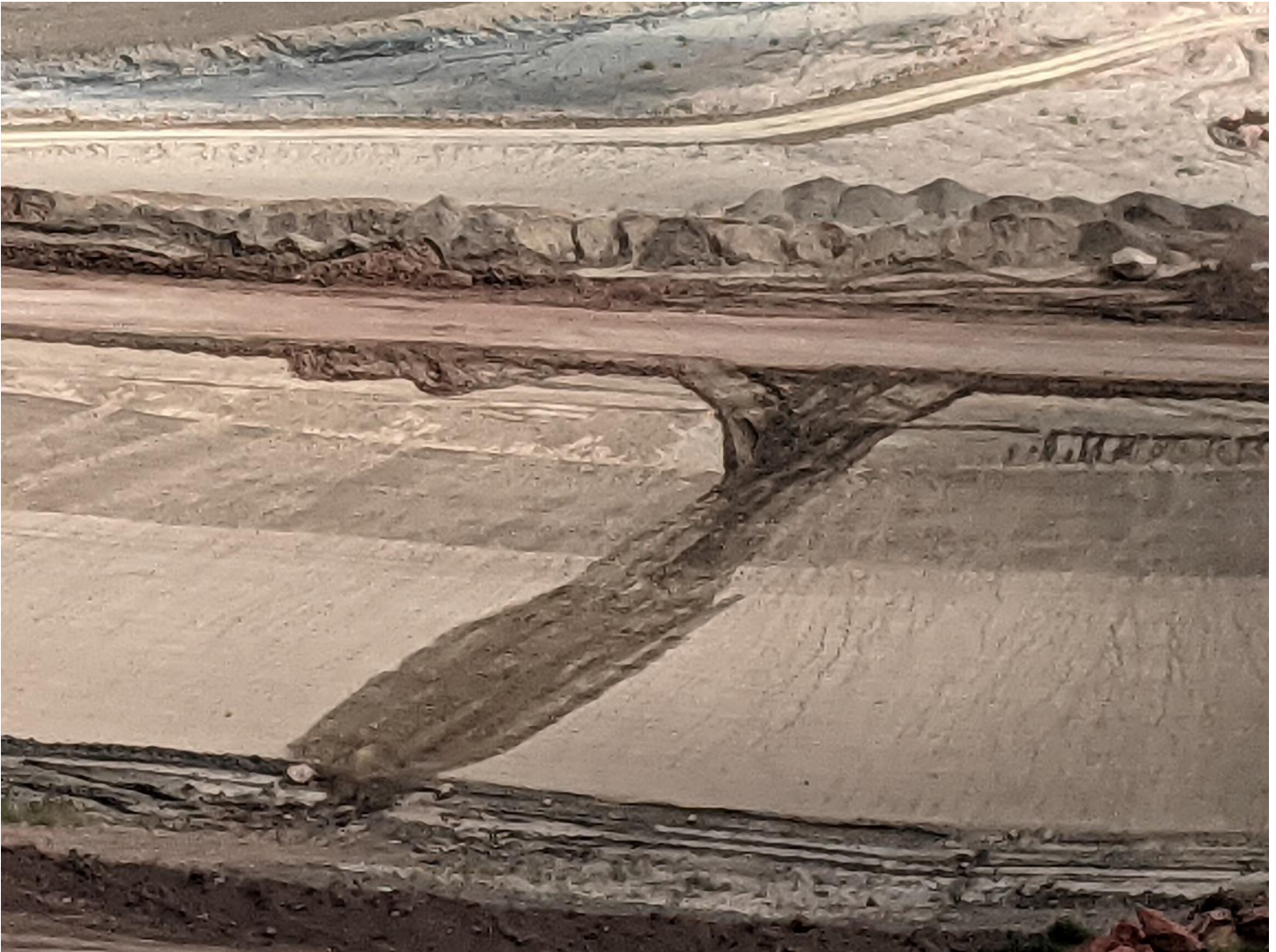
Gully repair along buttress slope.
