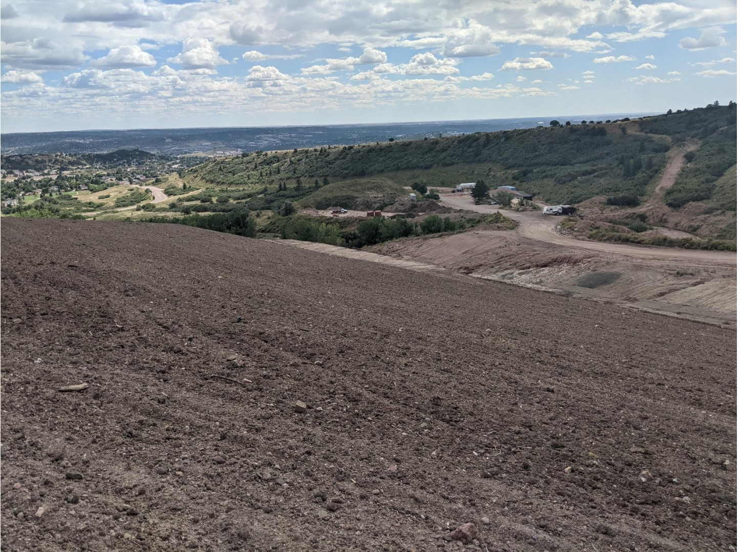
Northern slope topsoiled and benched for future trees.
