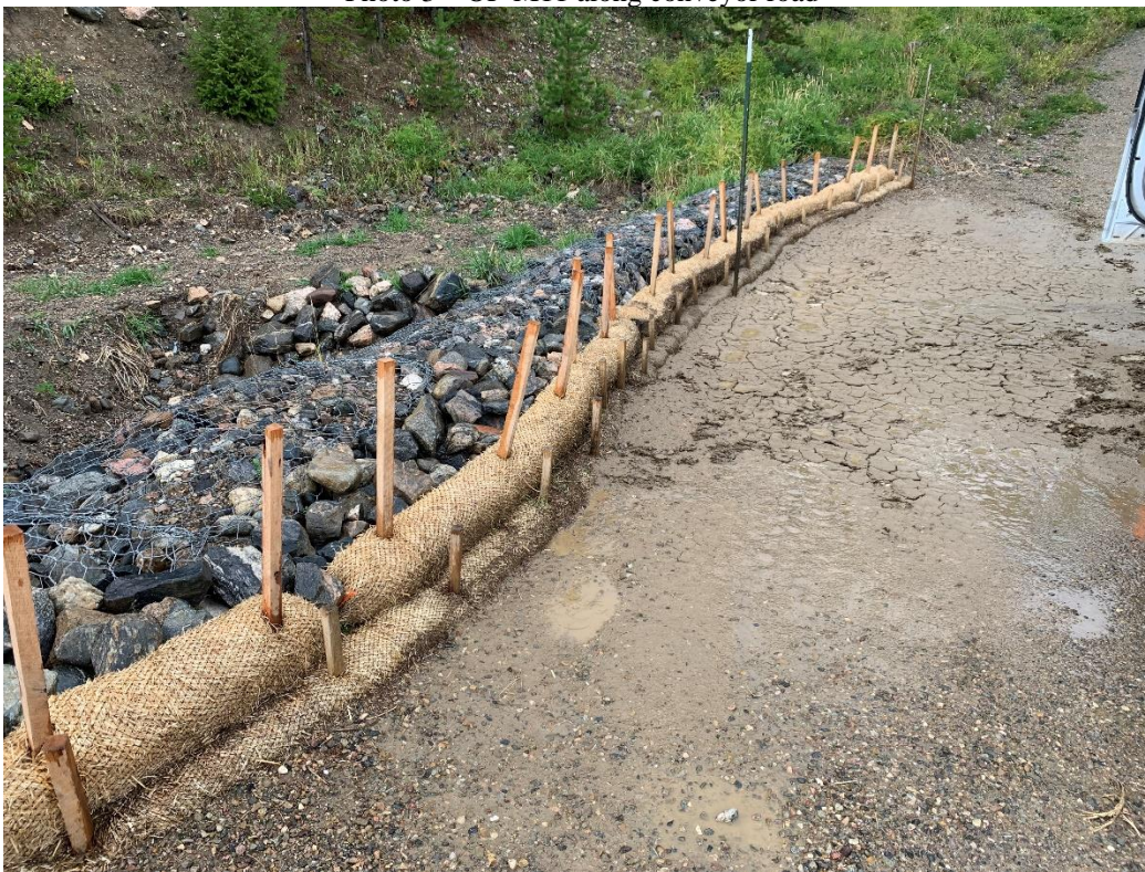
Photo 4 – OF-M5 has gabion cages create containment area.
