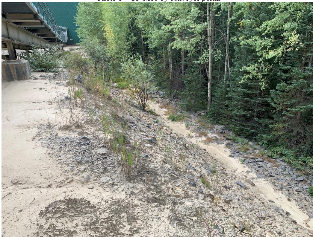
Photo 2 – Ditch at OF-M8 controlling dust from conveyor belt.
