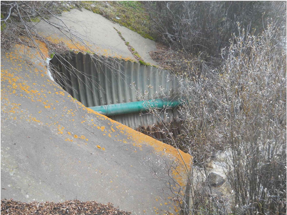
EXISTING CULVERT INLET - 2
