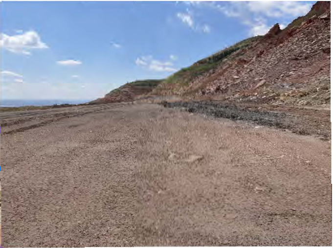
2. Compacted floor of first bench.
