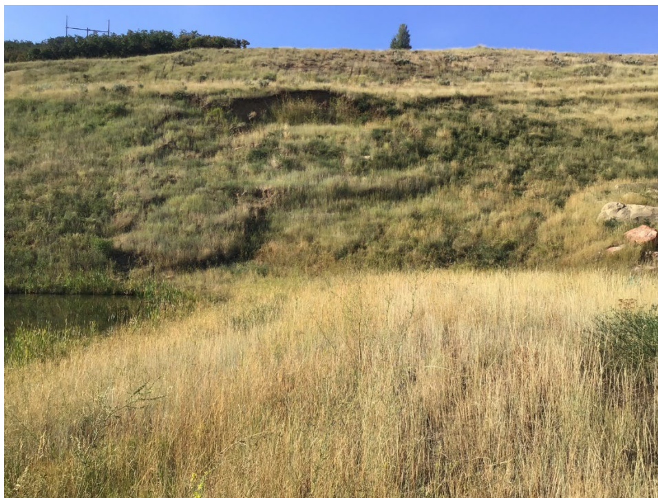
Photo 2: Slump above Pond 6.
