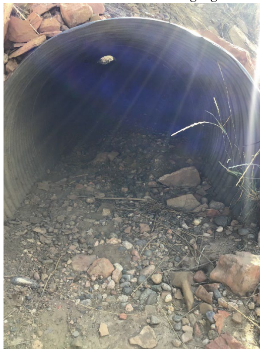
Photo 6: Debris in culvert on road above Pond 6.
