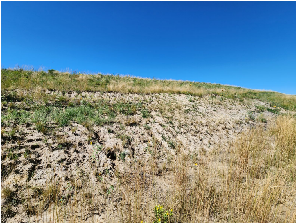
Photo 10. Eroded slope forming rills between phase 3 and phase 2 mining areas, looking southwest.
