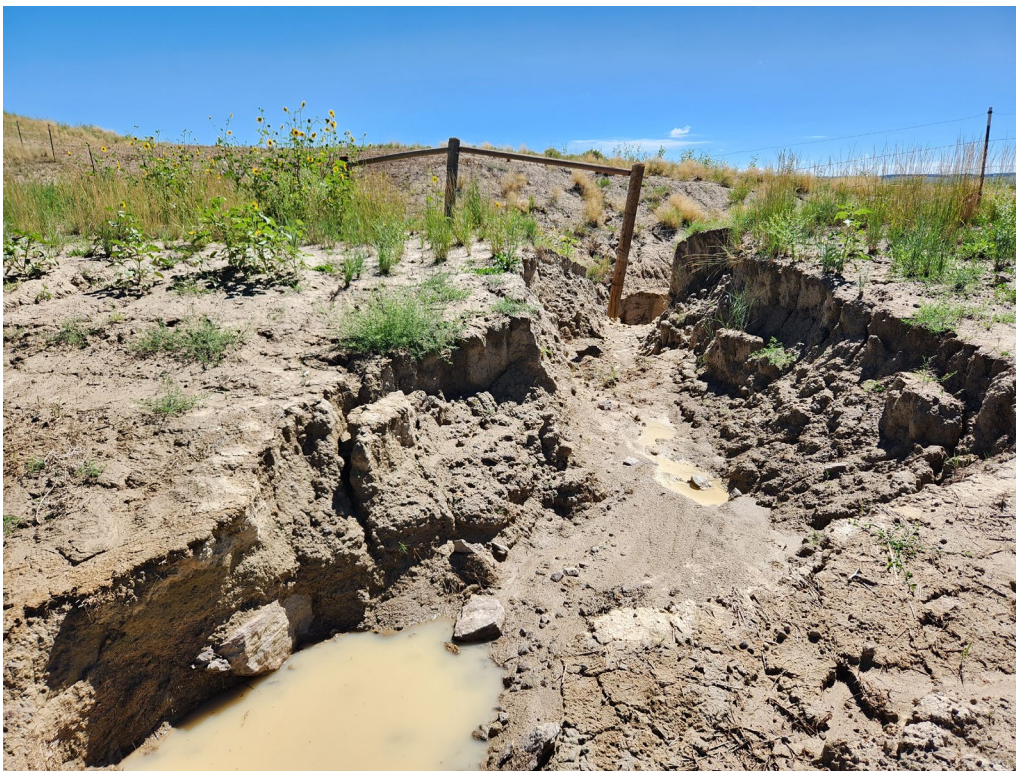
Photo 21. Gully leading from detention basin to natural drainage at eastern permit boundary, looking east.
