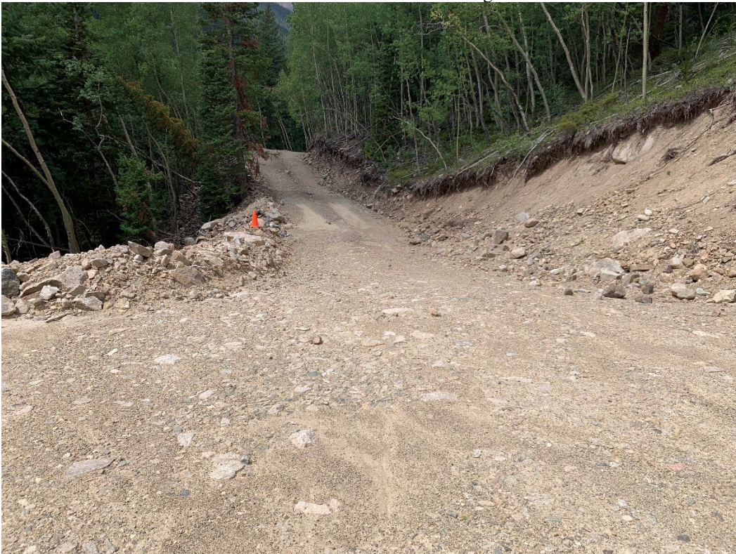
Photo 2 – The pad and access road with berm to control sediment
