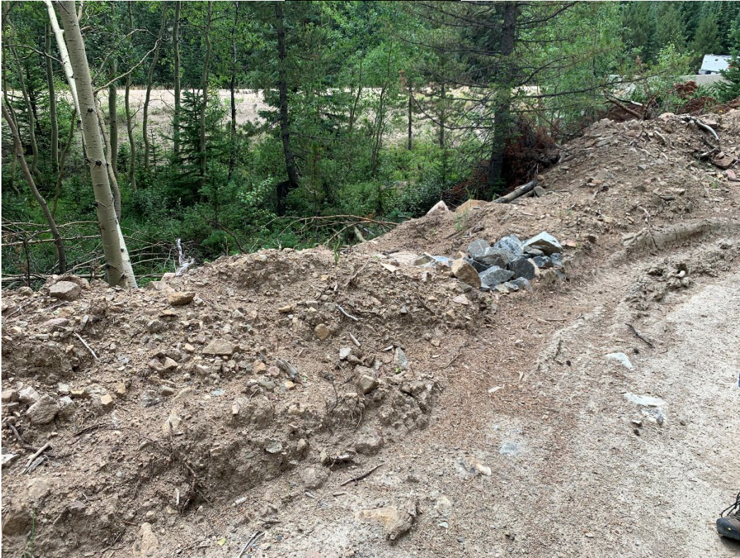
Photo 1 – Check dam at bottom of hill along access road
