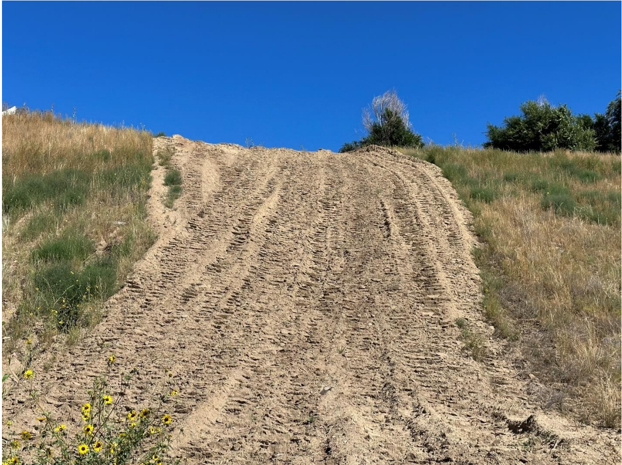
Photo 7. Recent repair on western portion of buttress
