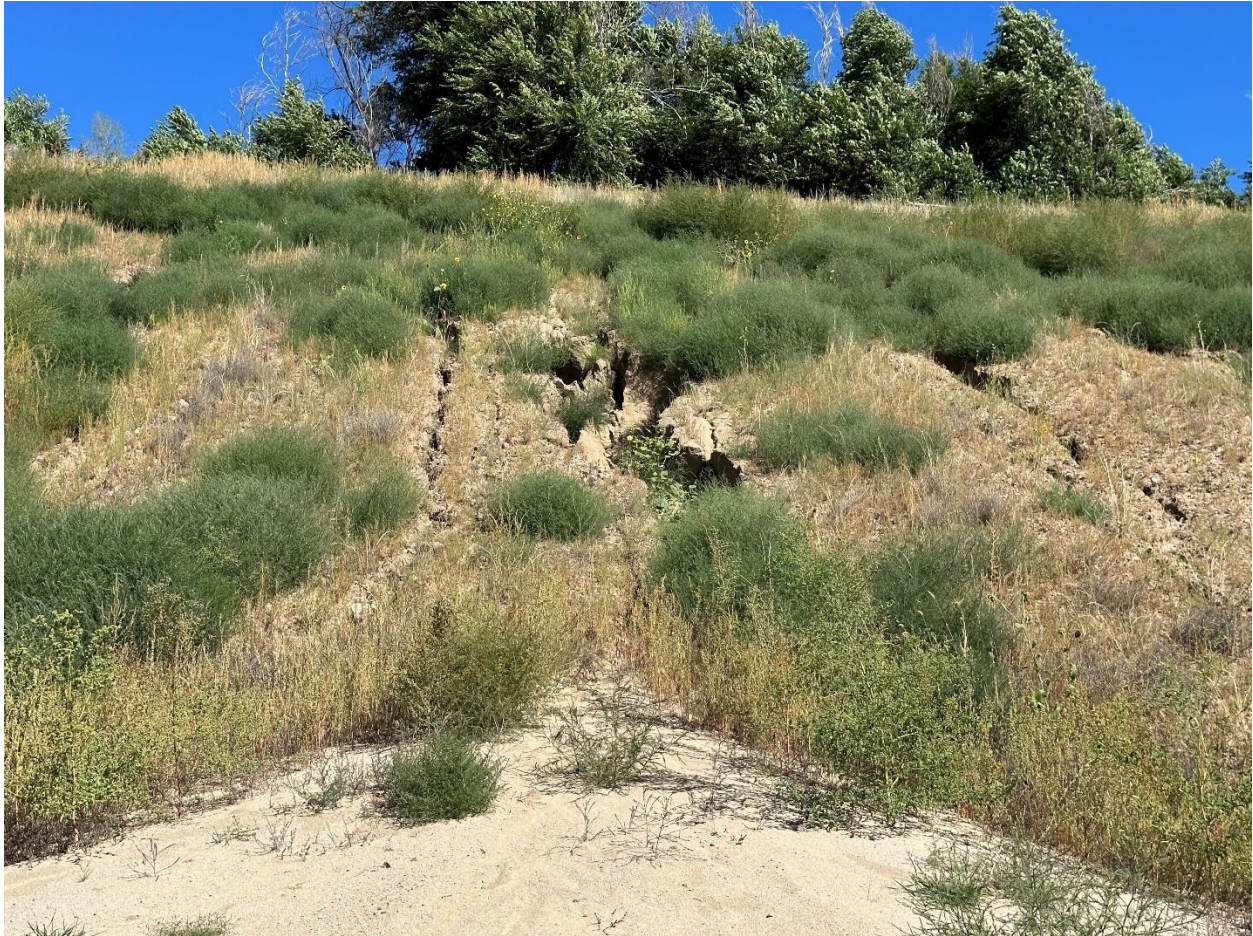
Photo 5. Erosion gullies in central area of buttress
