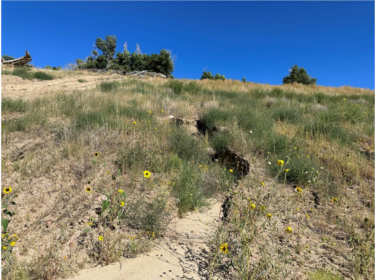
Photo 4. Erosion gullies in eastern portion of buttress
