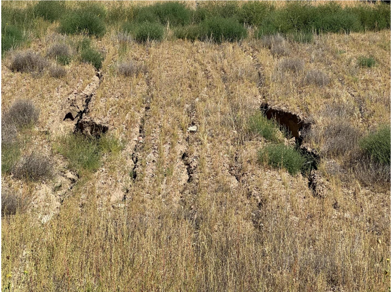
Photo 6. Erosion gullies in central area of buttress
