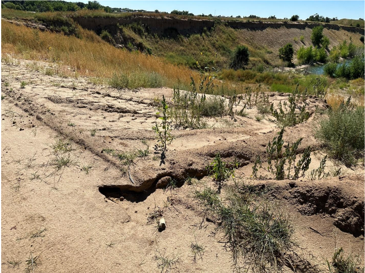
Photo 2. Erosion gully on ditch access road
