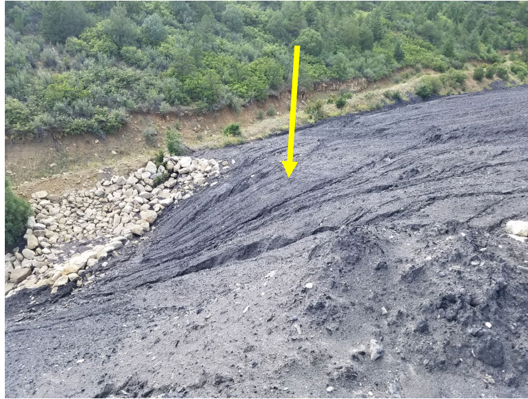
Figure 3. Rills forming on the western side of the upper bench of the RDA.
