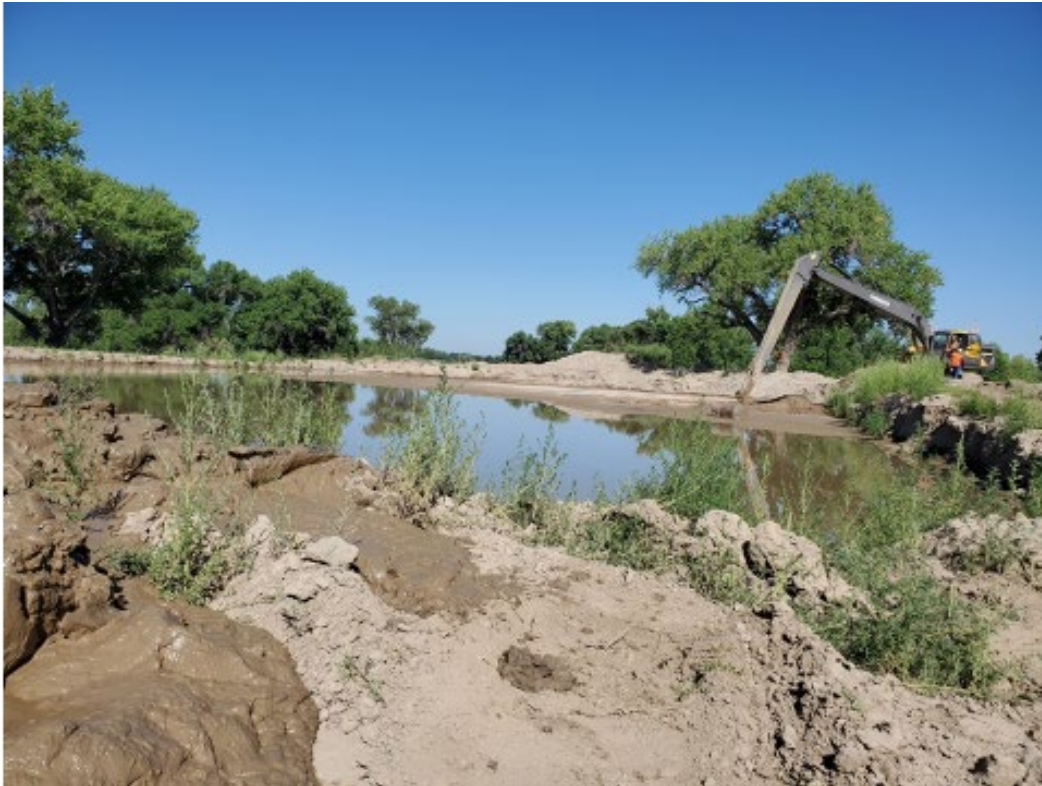
Photo 7: Looking north at the north pond. An excavator is removing the muddy waste and placing it along the berm separating the north and middle pond.
