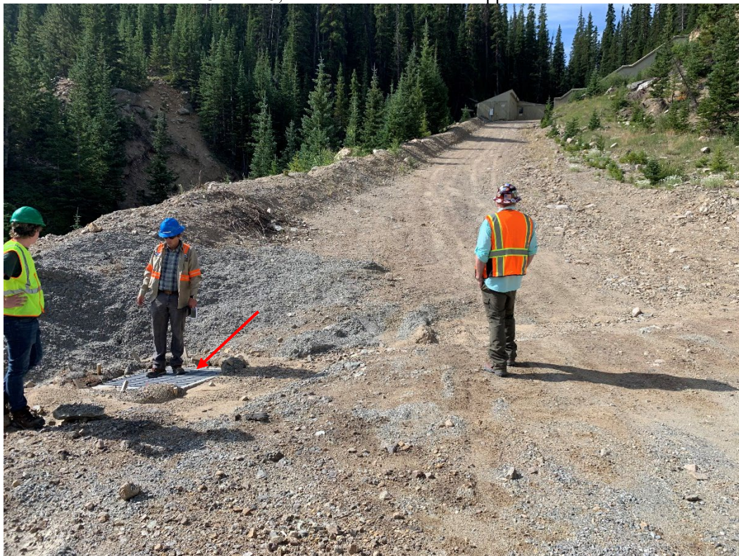
Photo 4 – OF18, buried vault box with grate top catches sediment.
