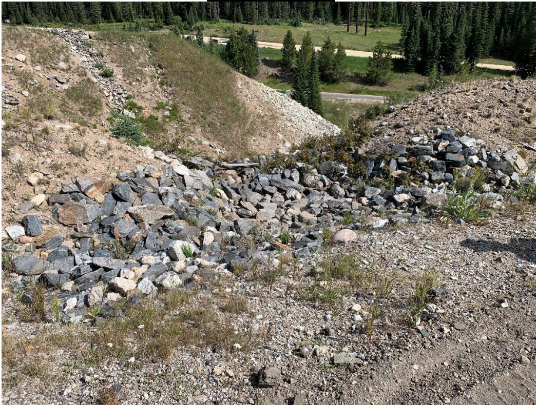
Photo 1 – OF7 check dam in working order.
