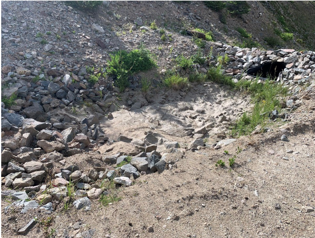
Photo 3 – OF15, clear of obstructions and appears stable.
