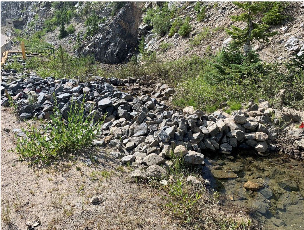
Photo 2 – OF8B, two check dams leading to Butler Gulch
