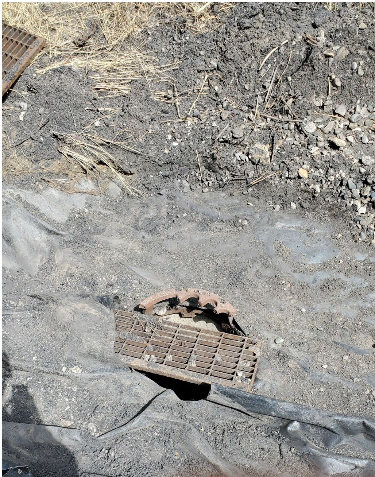
Figure 11: Drop inlet from D5E-1 into C5E-3
