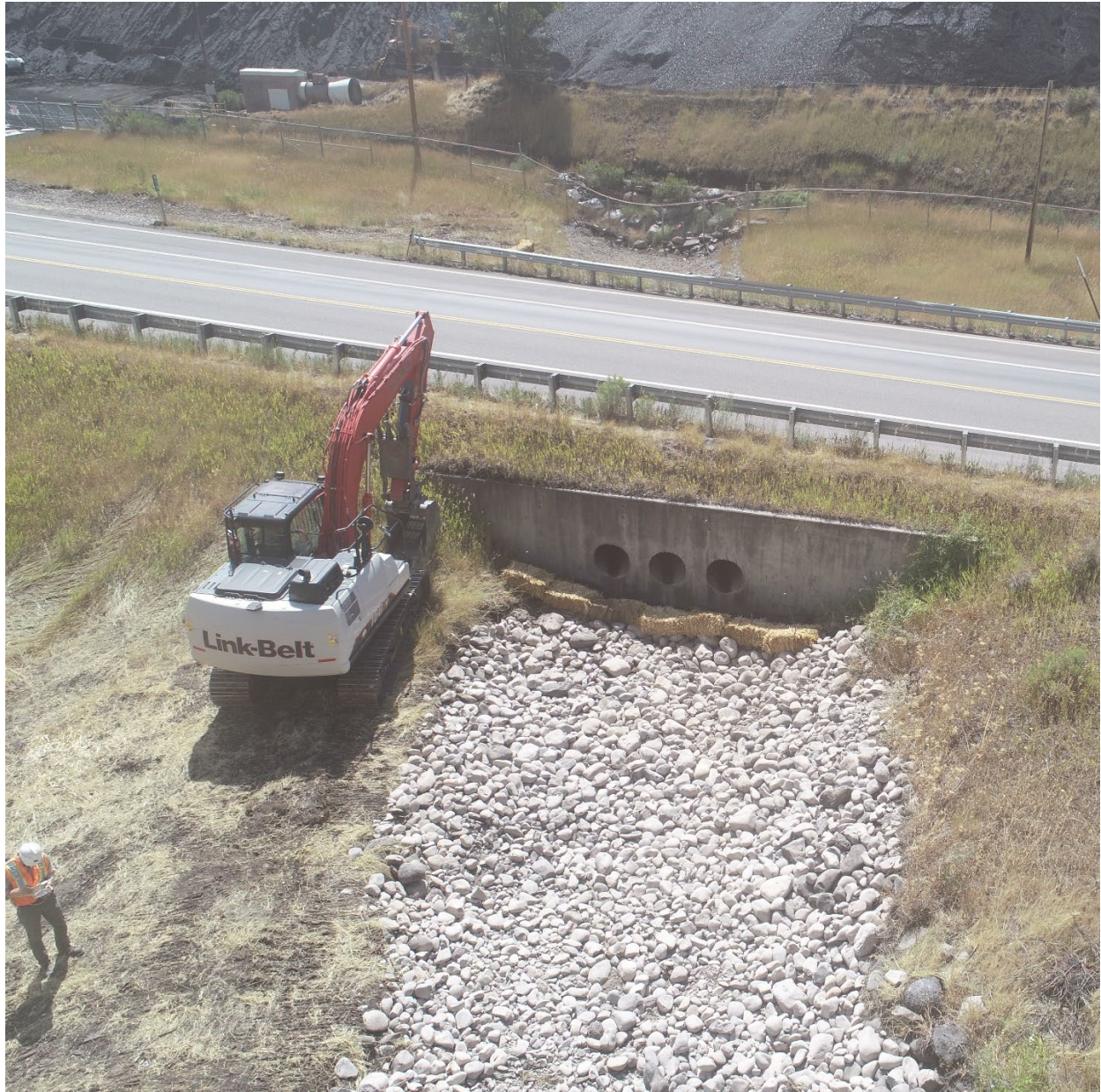
Figure 3: Drone image from north side of Highway 133 looking south, showing highway culverts with clean riprap and fresh straw bales
