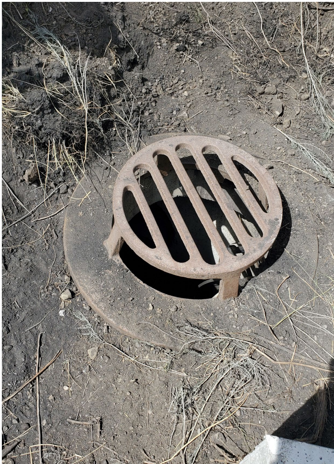
Figure 17: Grating above drop inlet from D5E-1A into C5E-3
