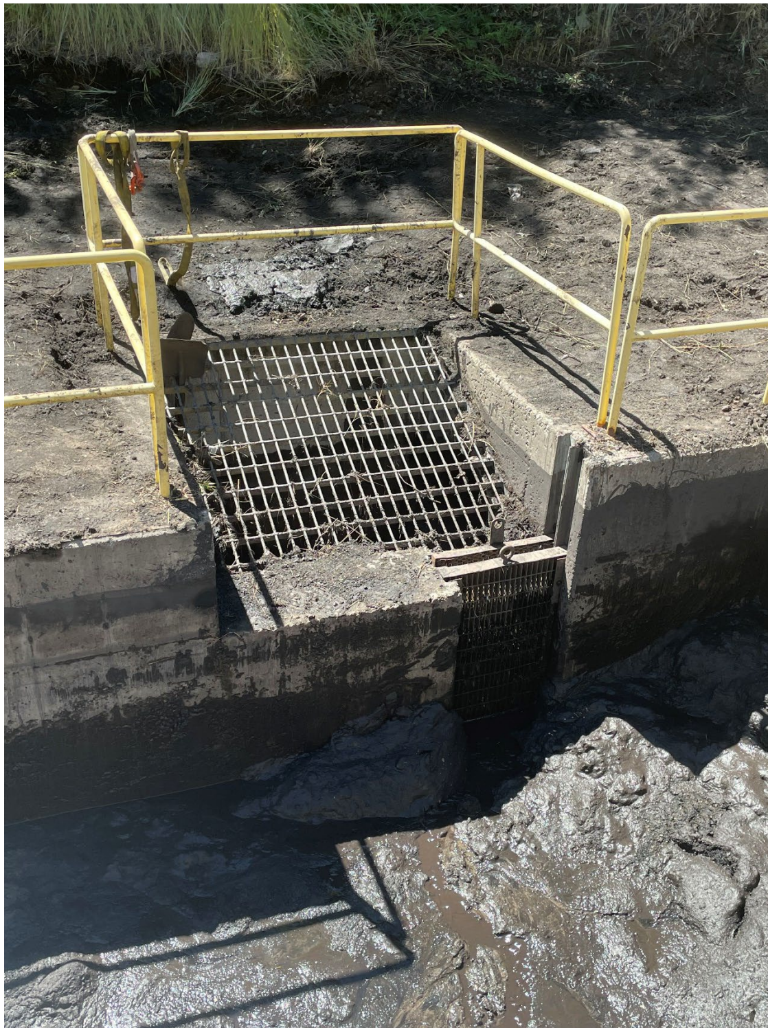
Figure 14: Sediment trap at outlet of C5E-2 following cleaning (1 of 2)
