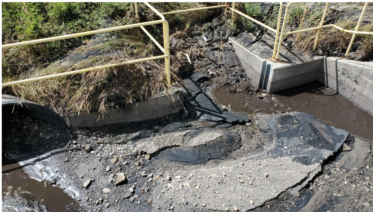
Figure 13: Sediment trap at outlet of C5E-2 (right), inlet of C5E-1 (left). Needs to be cleaned out.
