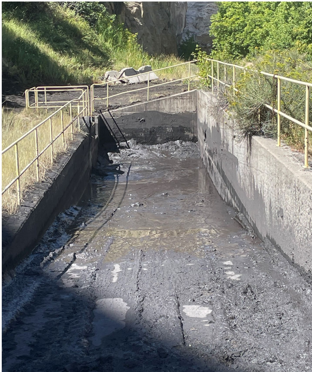
Figure 15: Sediment trap at outlet of C5E-2 following cleaning (2 of 2)
