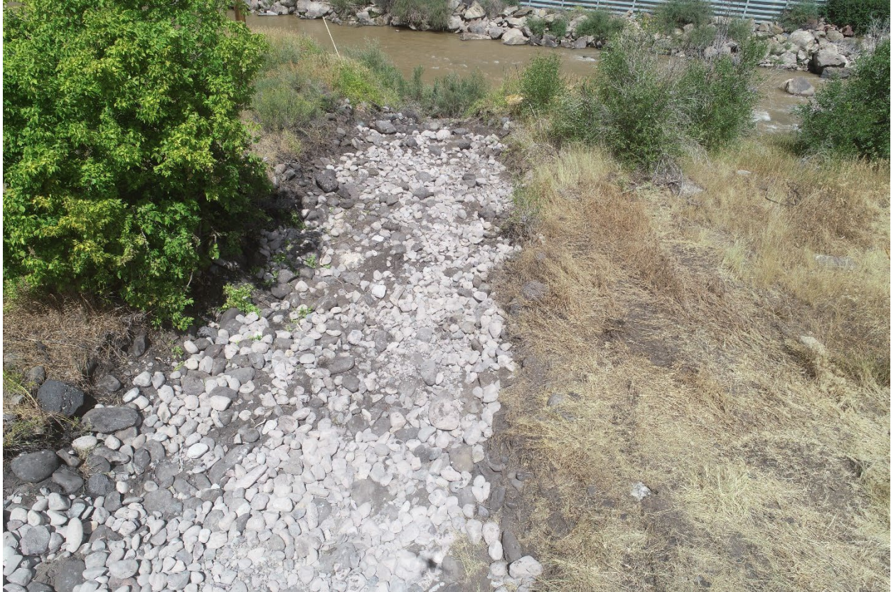
Figure 4: Drone image from north side of Highway 133 looking north, showing rip-rapped highway ditch leading to North Fork of the Gunnison River
