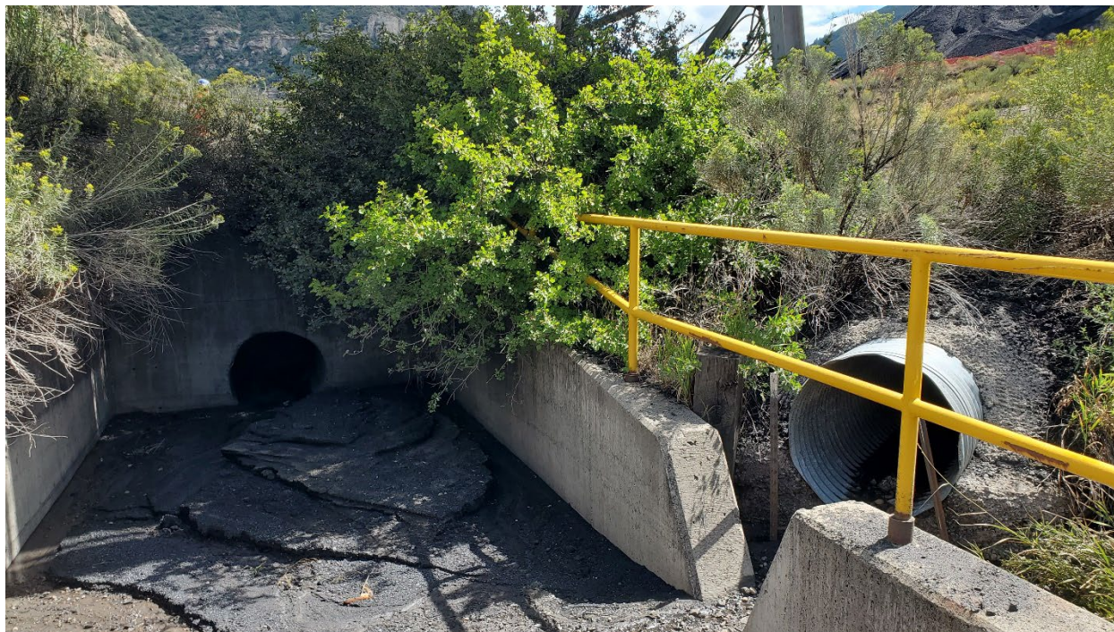
Figure 8: Sediment trap at C3-1A outlet/C3-1 inlet
