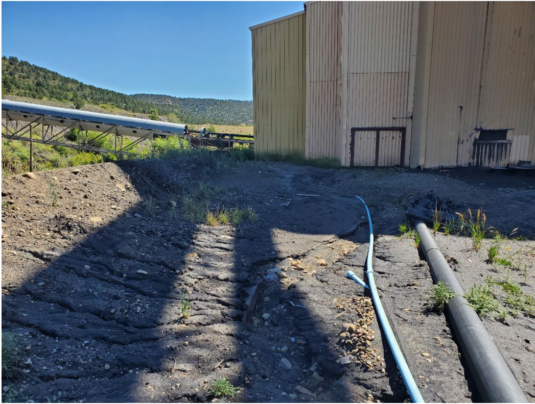
Photo 7 – Berm behind wash plant protecting the river
