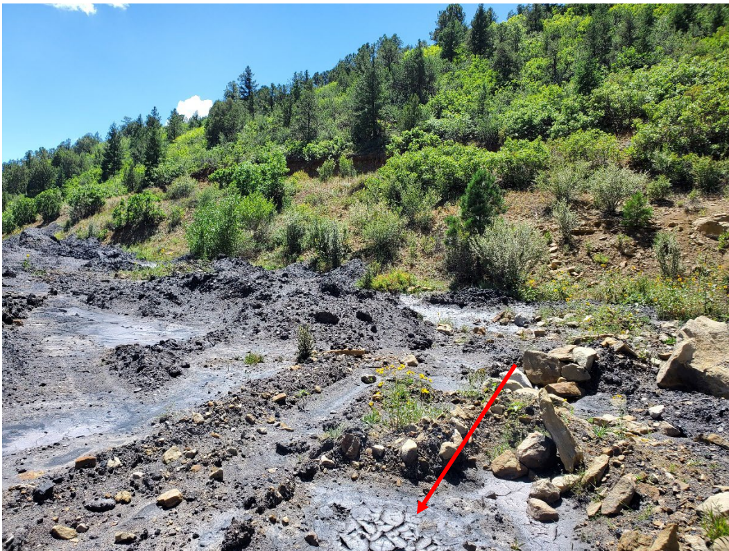
Photo 6 – Dried puddle on top of RDA shows water cannot drain properly.
