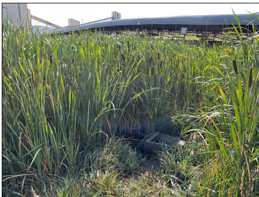
Photo 6: Weir at Pond D discharge, cattails provide additional water filtration.
