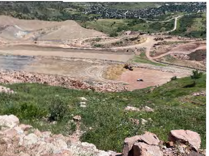
1. Offsite material placed and waiting for compaction.
