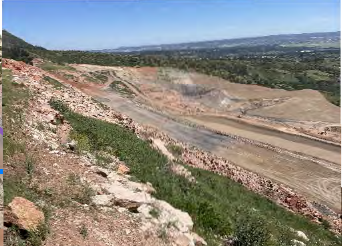
2. Compacted floor of first bench.
