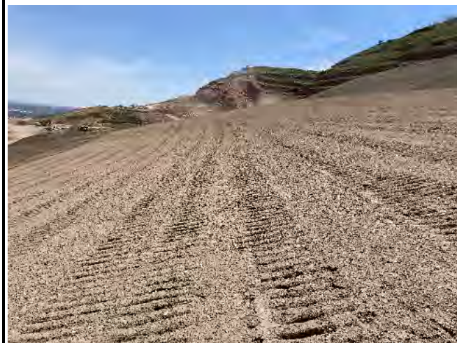
7. No cracking or slumping on bench slope.
