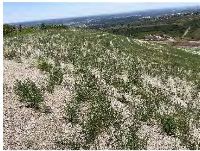
6. Vegetation growing within erosion blanket.
