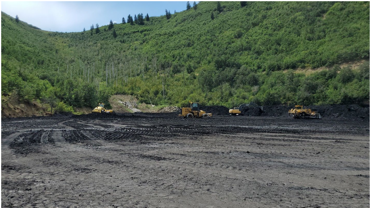
Figure 8: Compaction of refuse in progress on RPEE
