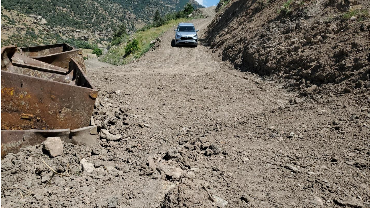
Figure 4: Surface water diversion at first hairpin
