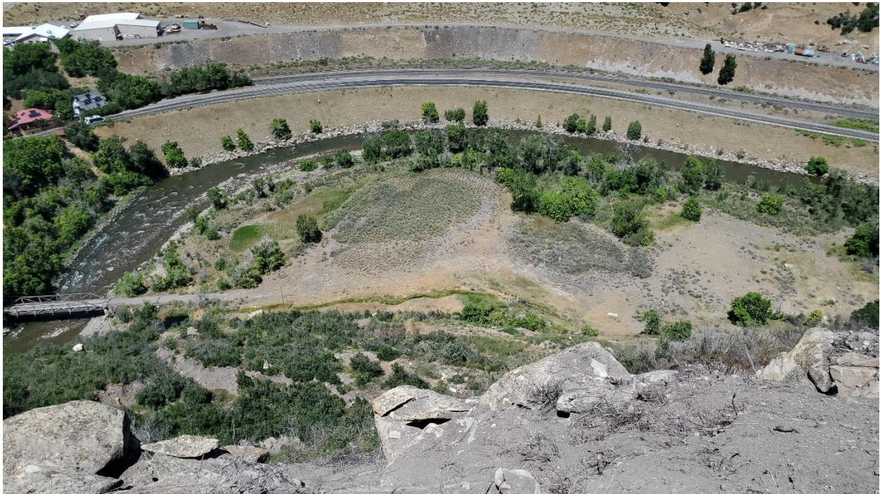
Figure 1: Overview of site from bench above slide
