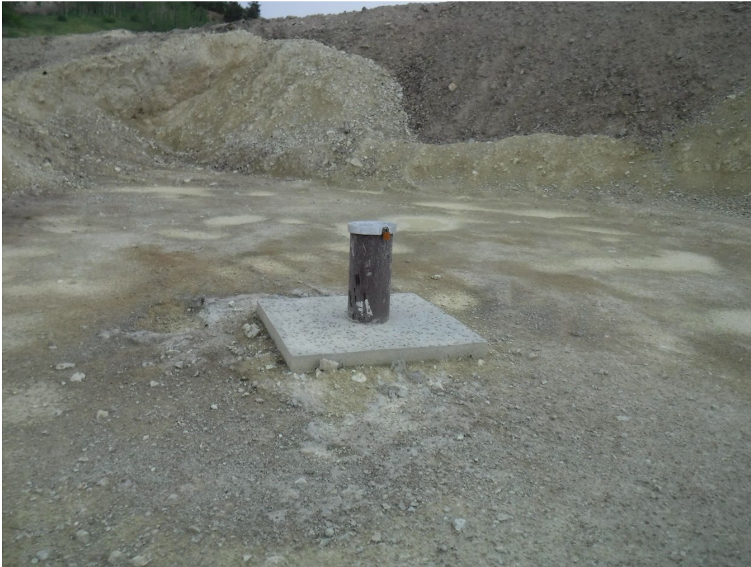
Photo 11: Newly installed Poverty Gulch POC well PGMW-5
