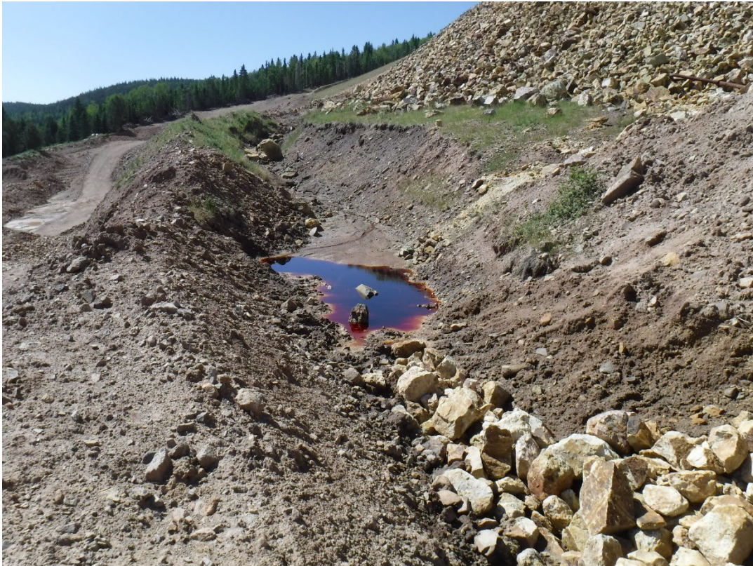
Photo 6: Looking south at the drainage ditch that is flowing north to Seep1
