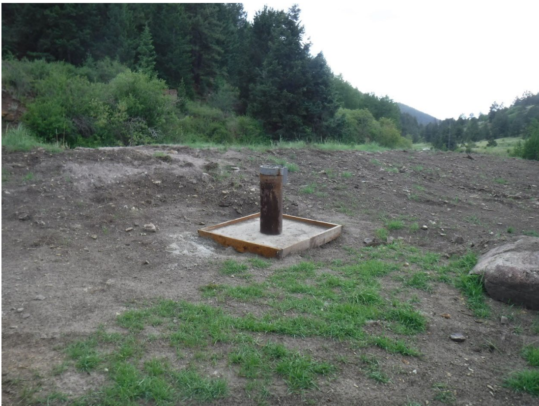
Photo 12: Newly installed Maize Gulch POC well SGMW-8
