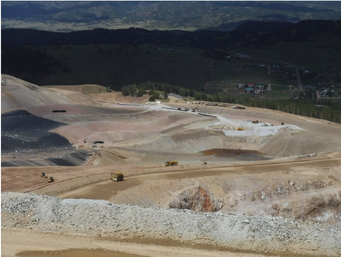
Photo 9: Construction activities near the PSSA
