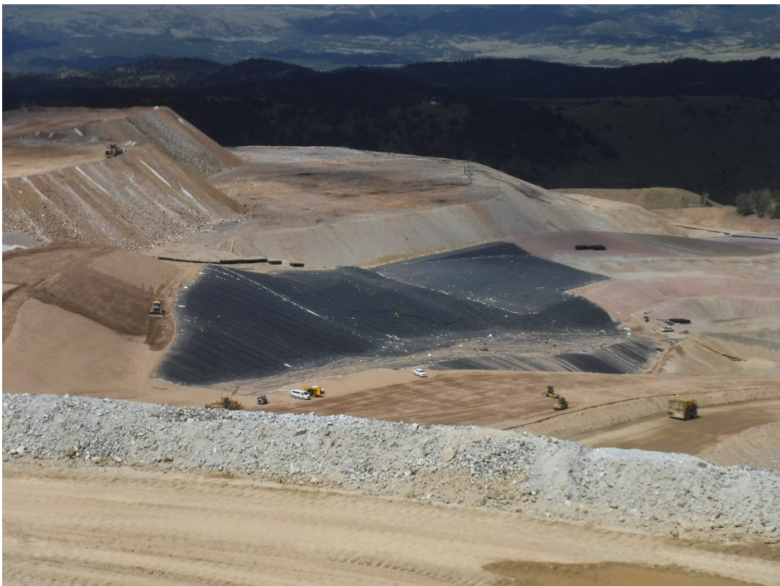
Photo 10: Geomembrane panel welding
