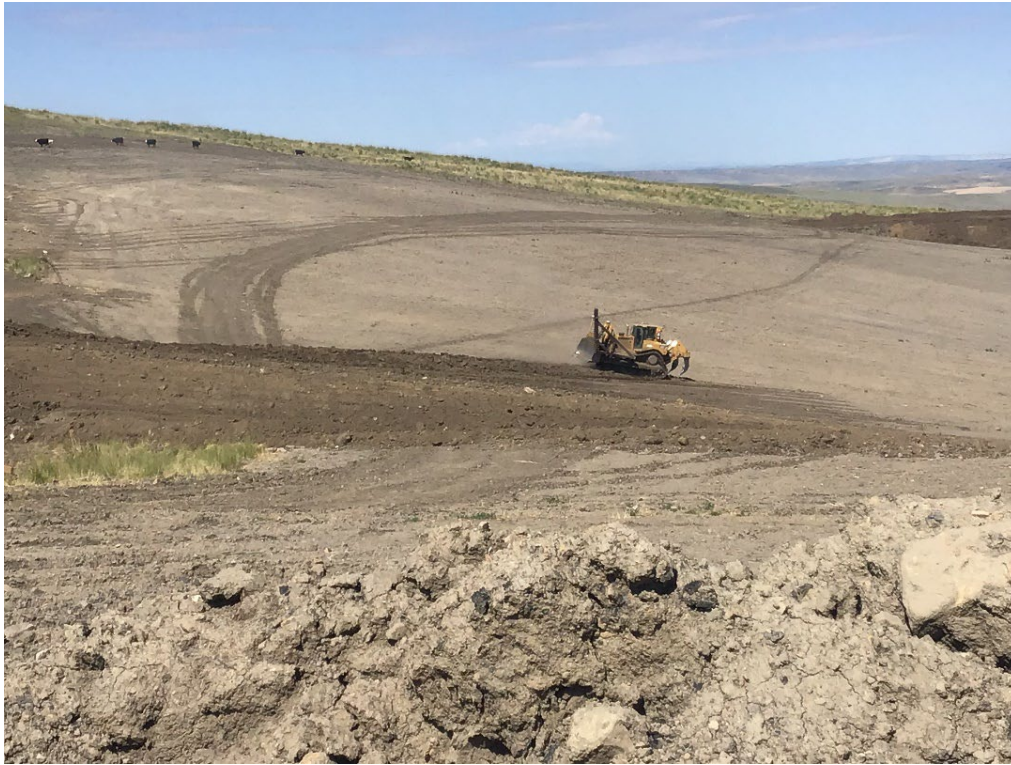
Photo 9: D Pit ripping and grading topsoil haul road.
