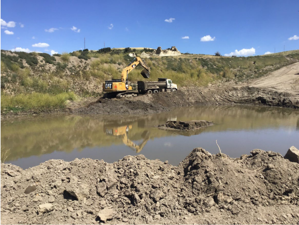
Photo 5: Dozer basin along main haul road undergoing dredging.
