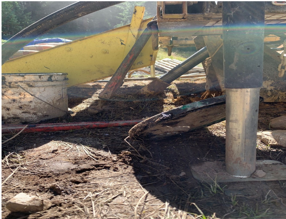
2. WP-10 borehole location with drill rig and HQ rod prior to abandonment
