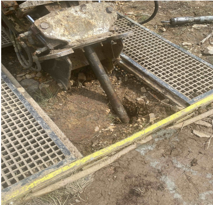
5. Cement injection head mounted on top of NQ rod
