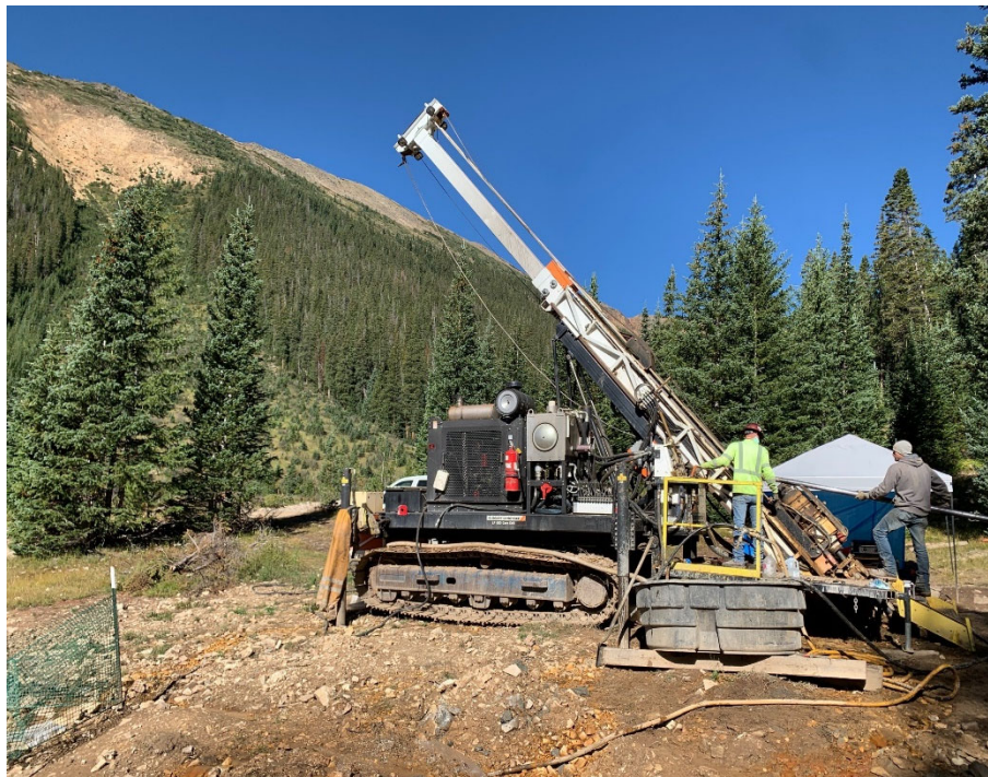
6. Drill Rig used to abandon borehole WP-10
