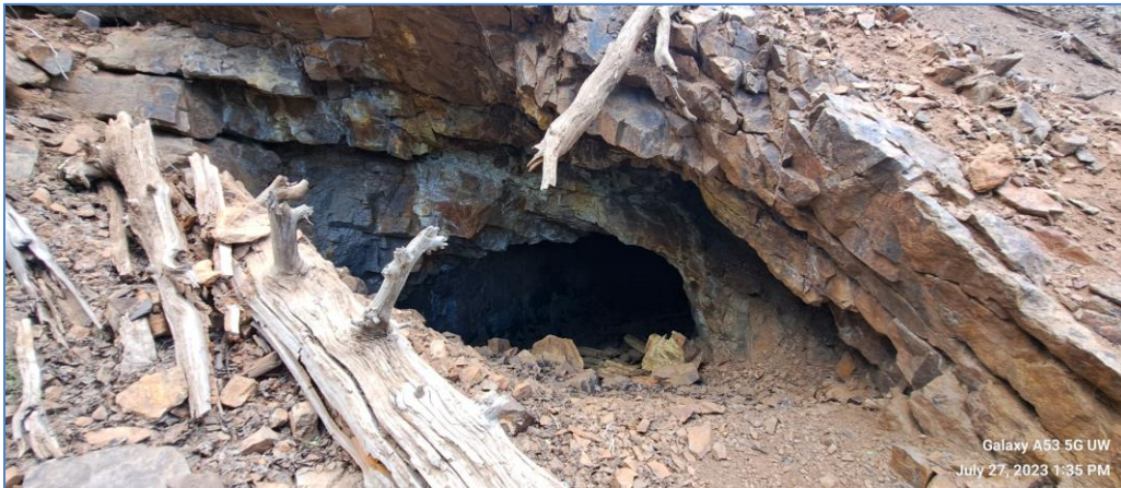
Figure 15: Partially Collapsed Adit (A). Location E on the map.
