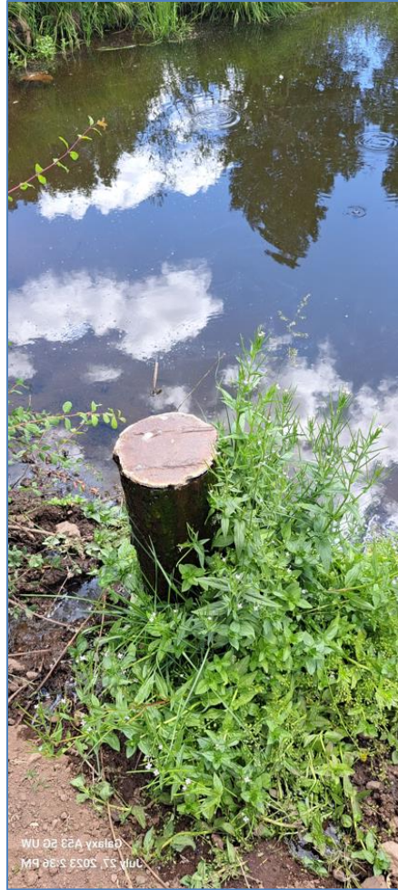
Figure 9: Stock pond located at hairpin in previous photo. There is what appears to be a leaking, capped off well or borehole casing that is seeping water out of the welded cap. Location D on map.
