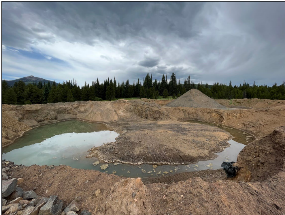
Photo 6: View inside the excavated area. All captured stormwater and snowmelt infiltrates back into the ground.
