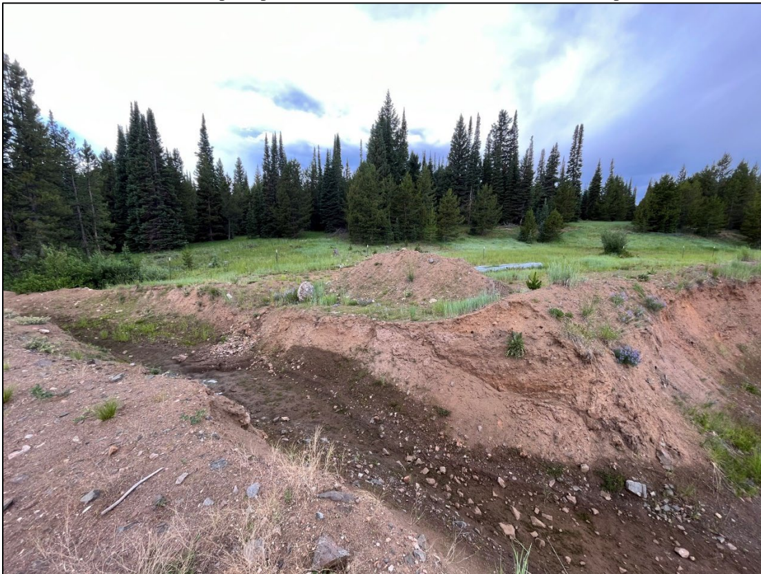
Photo 8: Water from the site is diverted through the stormwater berm and under the main entrance road.
