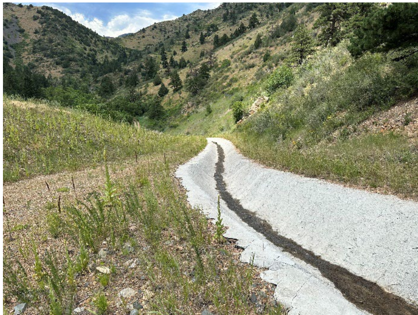
2. Stormwater Diversion Channel on the NWRP.
