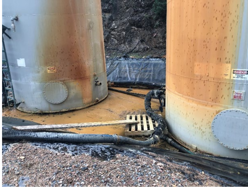
7. View of secondary containment for Backfill Slurry Tank and Reactor Tank.
