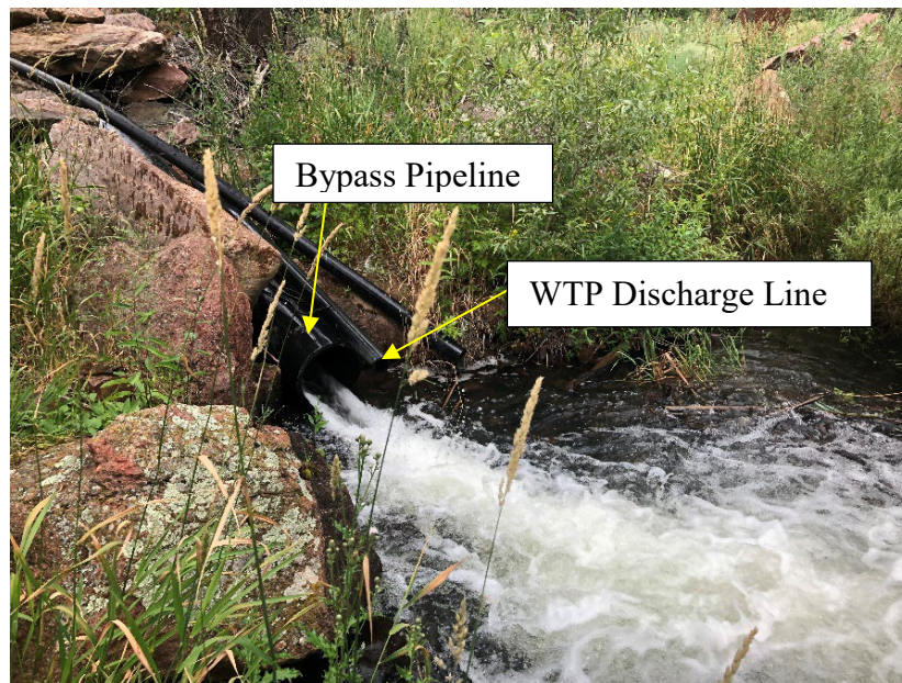
6. Bypass Pipeline discharging Ralston Creek Flows, no discharge from WTP.
