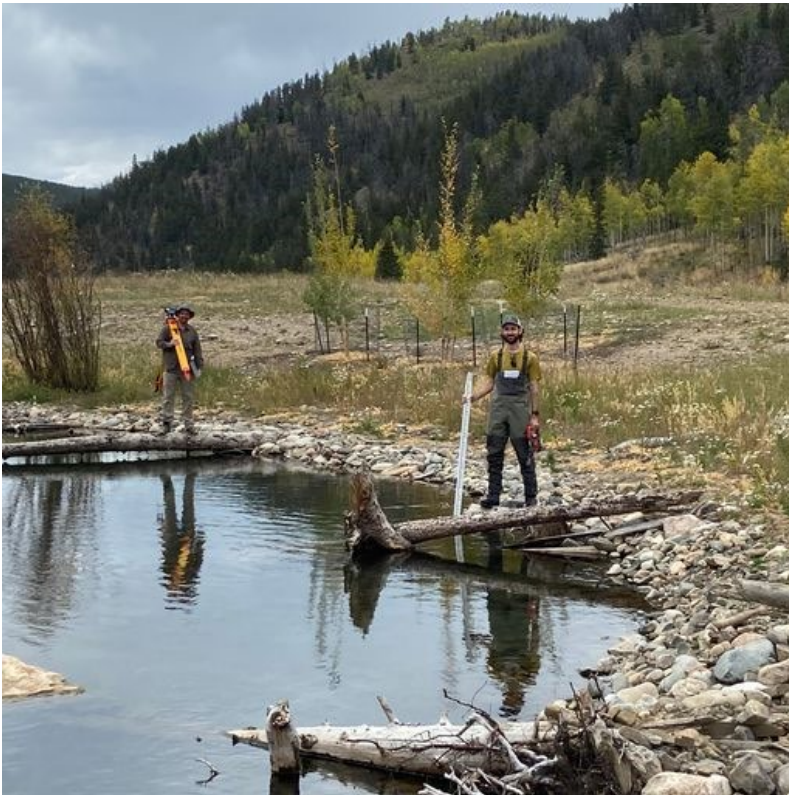
The newly constructed channel with willow and aspen plantings, large woody debris features, and revegetated uplands and riparian areas during initial site monitoring in the fall of 2022.
