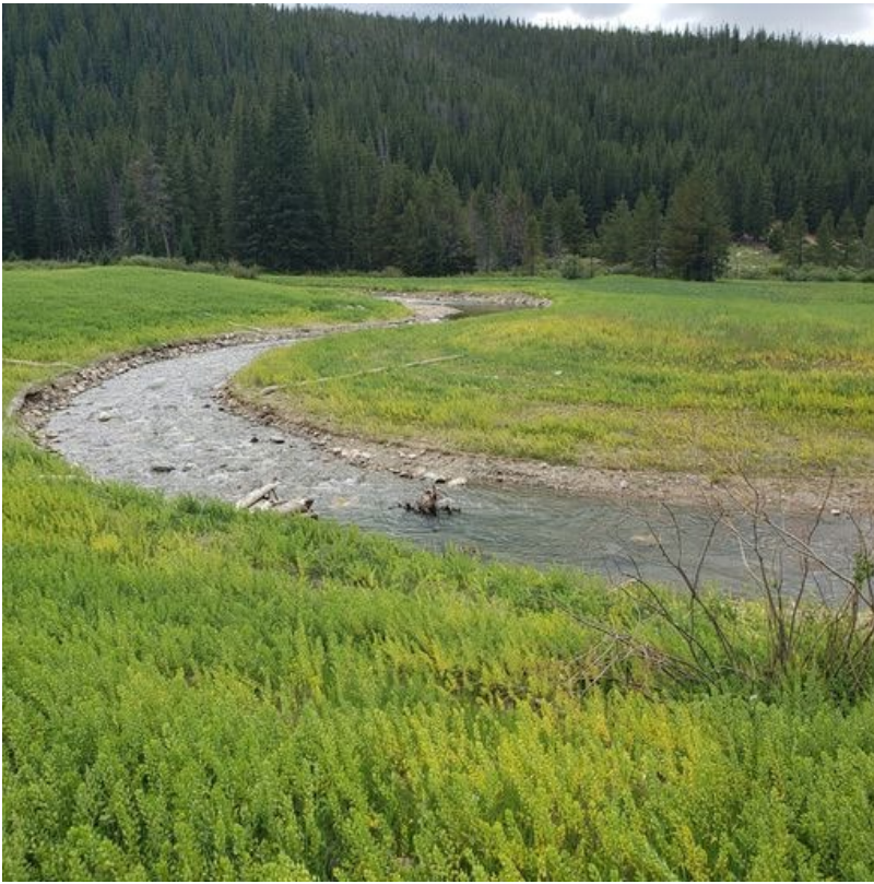
Typical cross valley view of the reclaimed permit area. Boulder features, large woody debris, riffles, and pool were installed in the river channel. Riparian and uplands were drill seeded with native grasses and planted with trees and shrubs.
