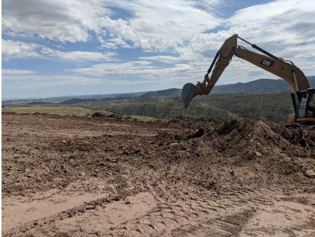
Topsoil stripping from Section 15 Pond.
