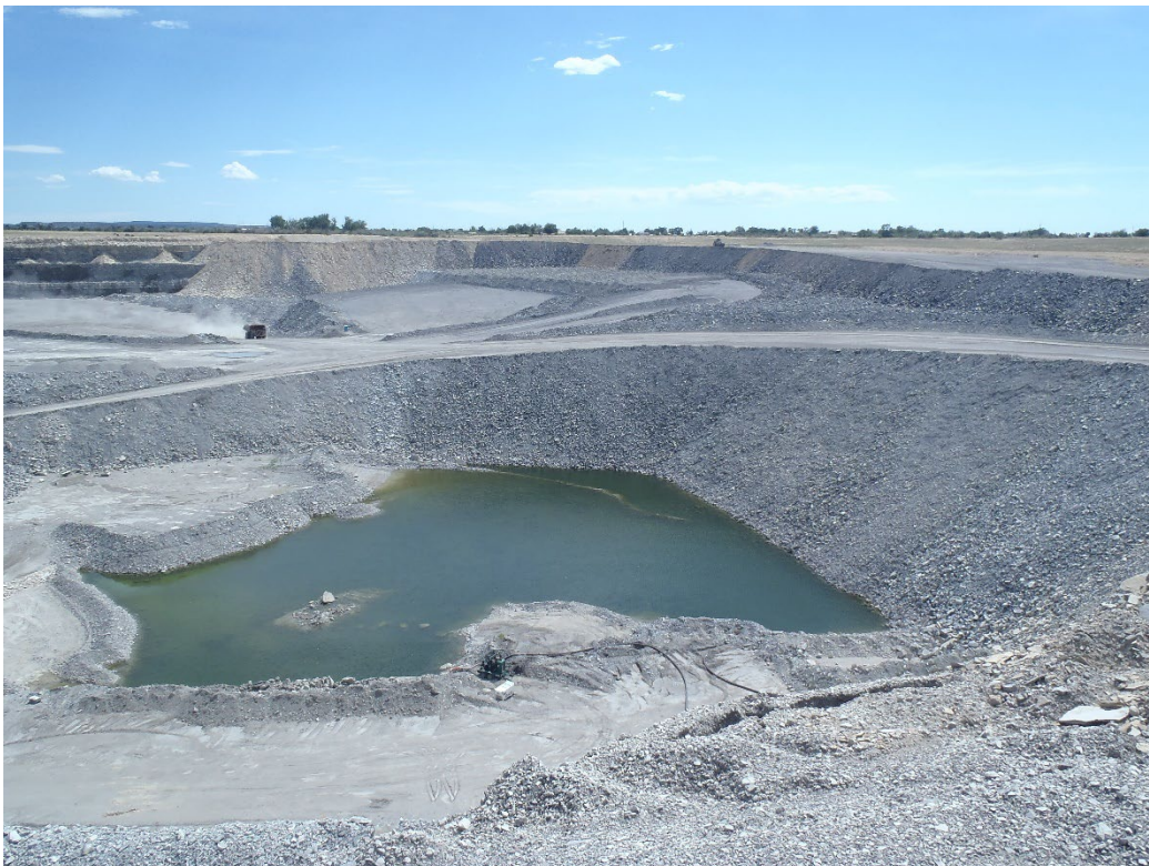
Photo 4. Exposed groundwater in active quarry (looking east).
