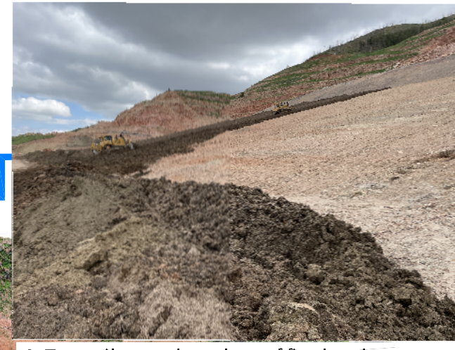
4. Top soil spread on slope of first bench.
