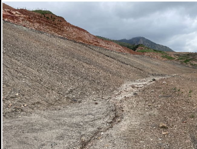
7. No cracking on buttress slope.
