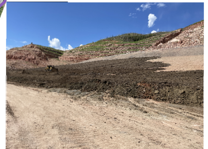
1. Top soil spread on slope of first bench.
