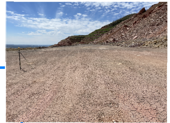
3. Compacted floor of first bench.
