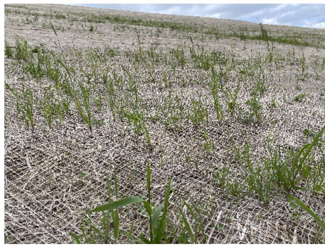
6. Vegetation growing within erosion blanket.
