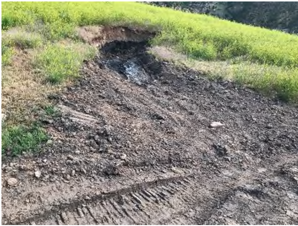
Photo 11 (left) view upslope (northeast) at the blowout and the former mudflow fan that has been mostly removed. Photo 12 (right) is a close-up view of the cover soils and gob material in the blowout headwall.
