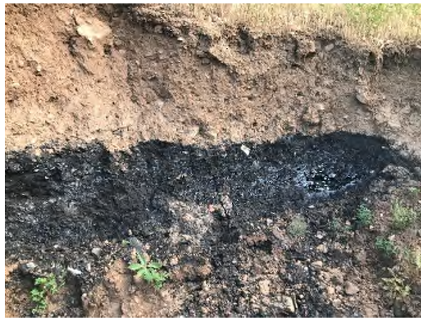
Photo 11 (left) view upslope (northeast) at the blowout and the former mudflow fan that has been mostly removed. Photo 12 (right) is a close-up view of the cover soils and gob material in the blowout headwall.
