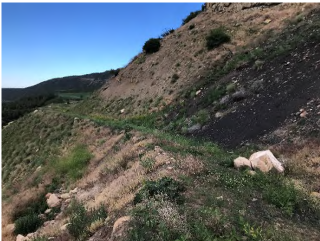
Photo 10. View west at the drainage ditch at the base of the hillside north of the gob pile. This is the uppermost drainage feature. It appears to be mostly intact (although it has some infilling and rockfall) and functions to drain snow and runoff around the gob pile.
