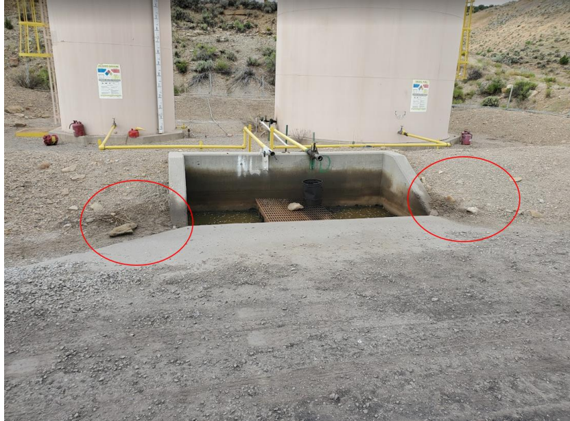
Photo 5: View to the southwest of fueling station. A small amount of diesel contaminated soil can be seen on the edges of the containment structure.
