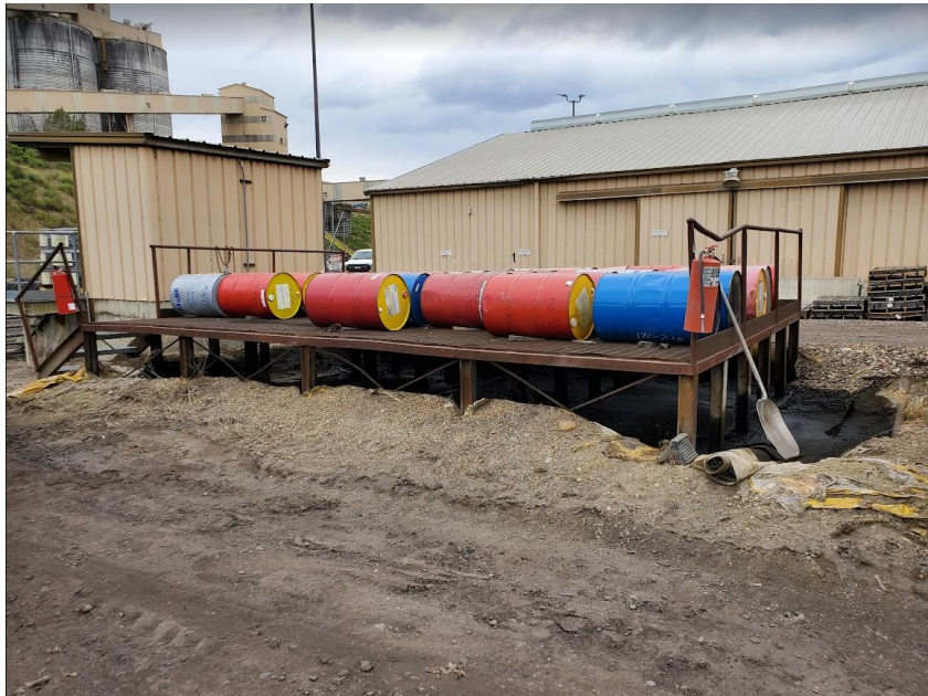
Photo 4: View to the southwest of 55 gallon barrels above secondary containment.
