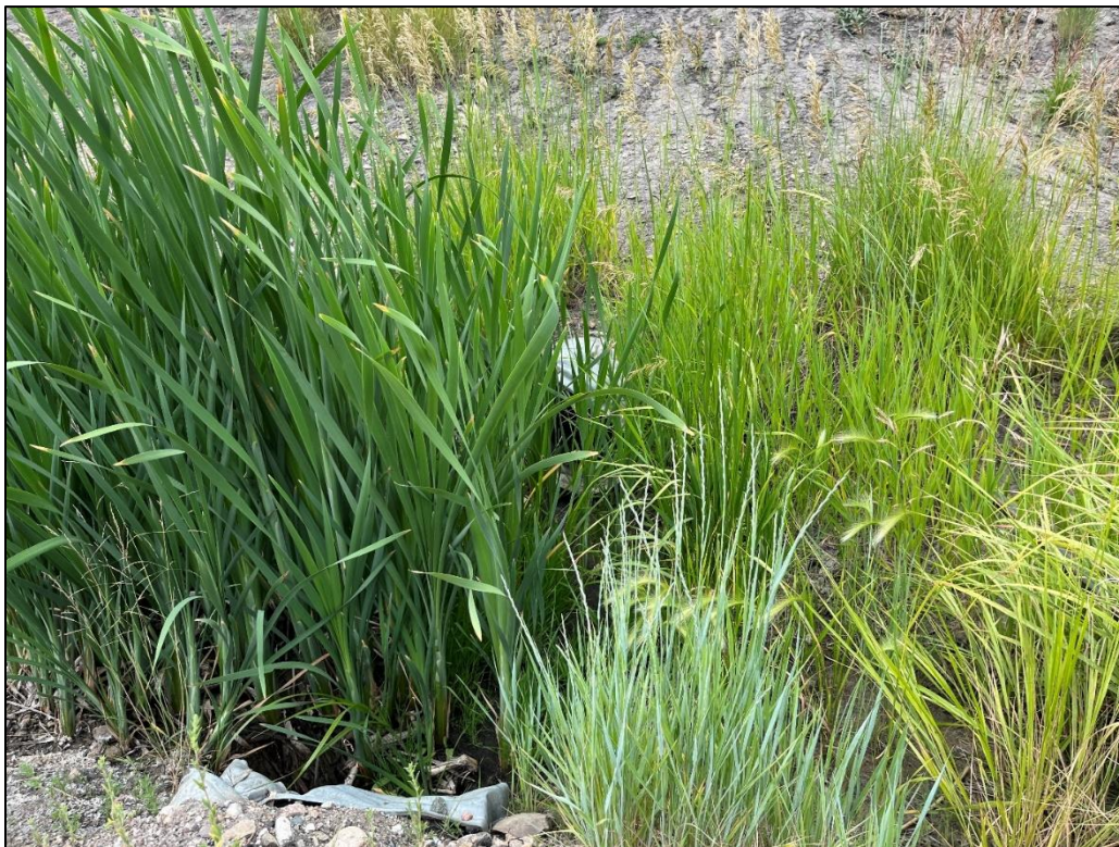
Photo 8: Culvert for Pond C, in need of cleanout.
