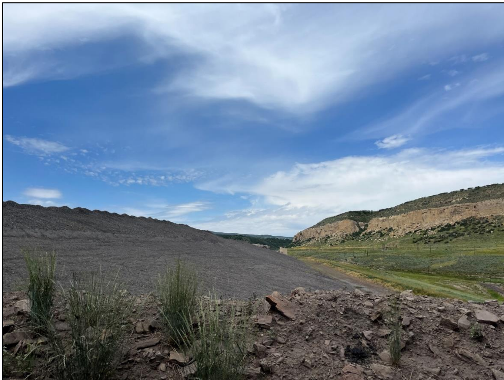
Photo 14: View West of the refuse pile, 2 nd lift (shown) is compacted and ready to be seeded this season.
