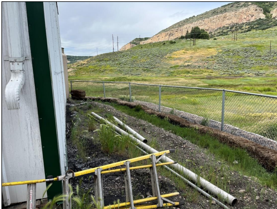
Photo 6: View of the back of the stoker coal loadout building, three ditches have been built to maintain water leakage while the building waits to be sealed.
