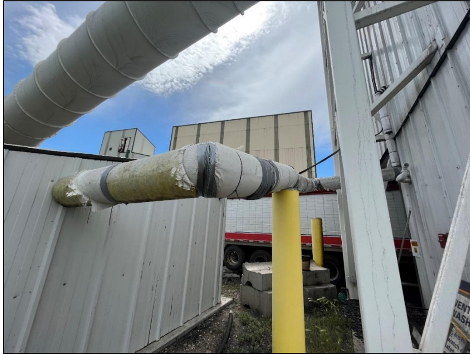
Photo 7: The main supply of water from the stoker coal wash plant operation drains through this pipe into a sump building adjacent.
