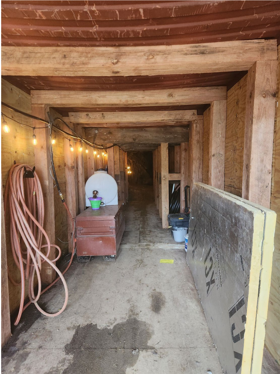
First container. Additional timbering to be added to create a box beam.
