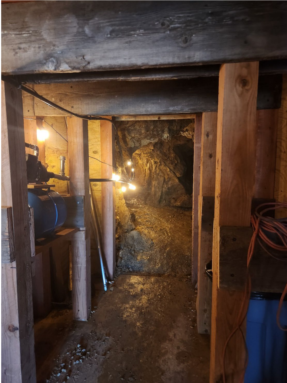
Second container with narrower timber span. Jet pump shown in photo.
